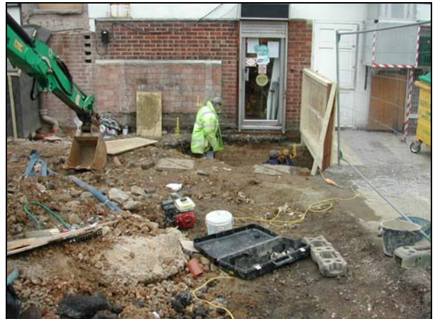
Plate 4: State of site from the south (30/1/06)
