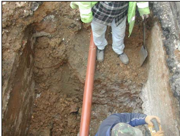
Plate 3: details of footings on the north side of the existing building
