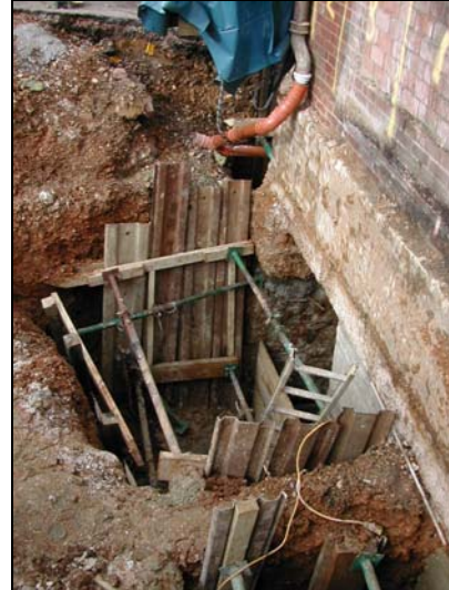
Plate 2: Detail of underpinning
