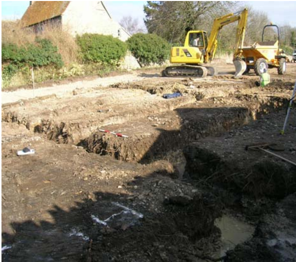
Plate 1: View of footing trenches for plot 1, looking northeast
