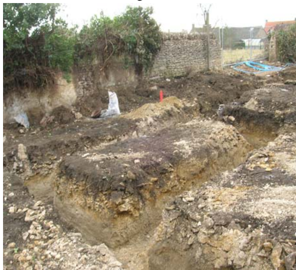
Plate 3: View of footing trenches for plot 2, looking southwest
