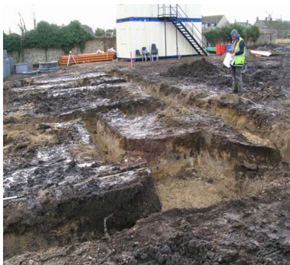
Plate 5: View of plot 3 footing trenches, looking southwest
