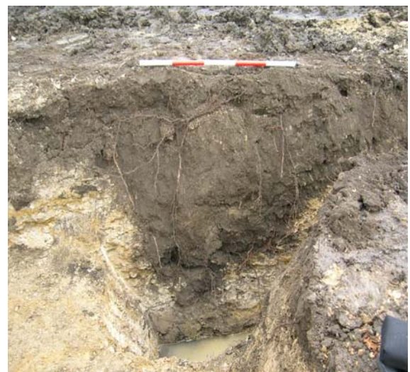
Plate 6: South facing section of plot 3 footing trenches, showing a modern, topsoil filled feature
