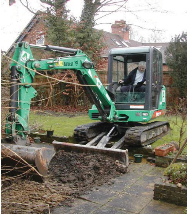
Plate 1: View of trench 1 during excavation
