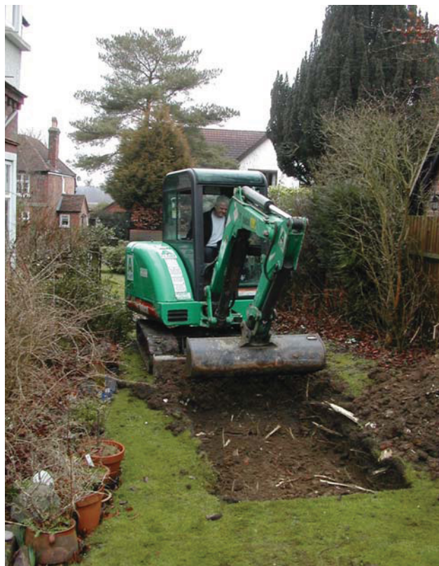
Plate 3: Removing topsoil in trench 2
