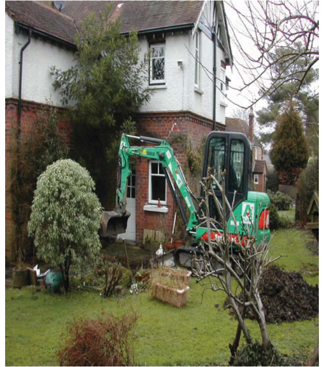
Plate 2: View of trench 2 during excavation
