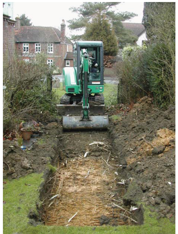
Plate 4: Trench 2 showing of root action
