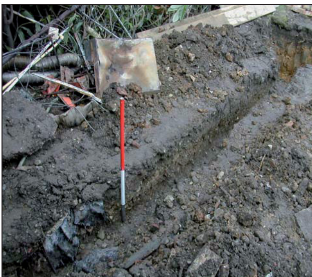
Plate 5: Detail of the service trench
