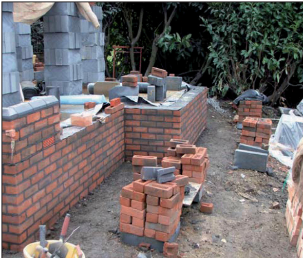
Plate 3: Detail of the constructed footings for the northwestern extension
