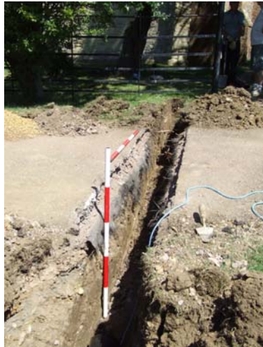
Plate 1: Trench crossing footpath toward church
