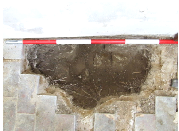
Plate 6: Sub-angular limestone foundation blocks at the base of excavation within the church.
