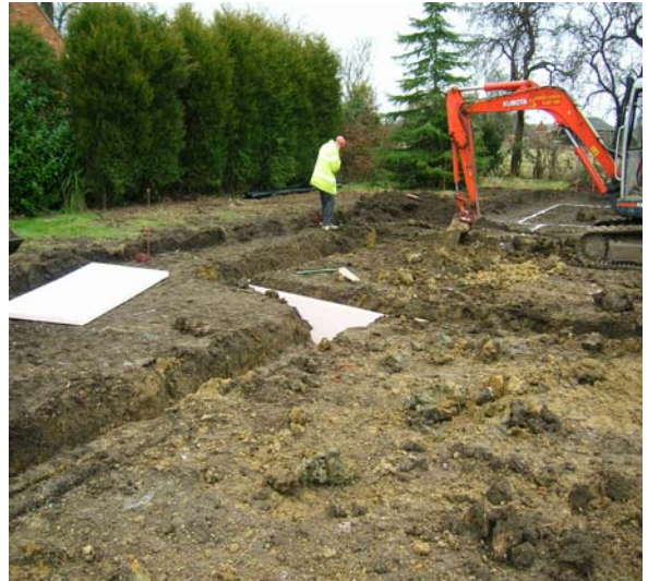
Plate 2: View of the site during excavation of the footing trenches
