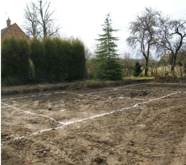
Plate 1: View of the site prior to excavation of footing trenches
