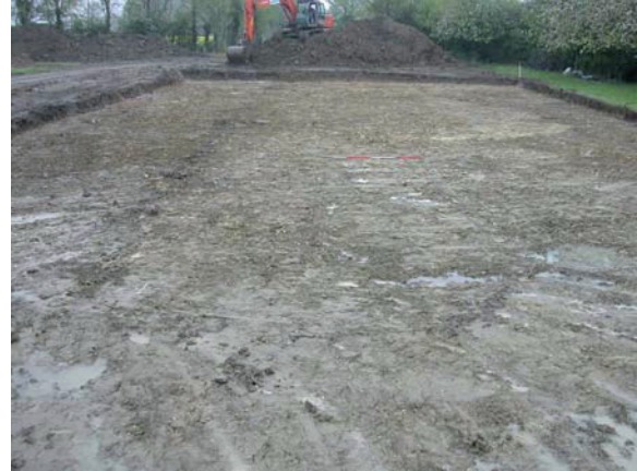
Plate 2: General view north of stripped area
