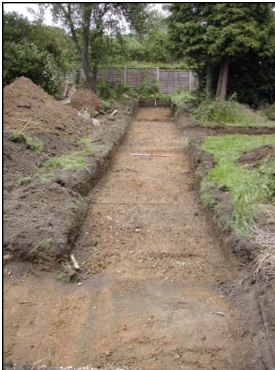
Plate 3: Trench 3, looking north east
