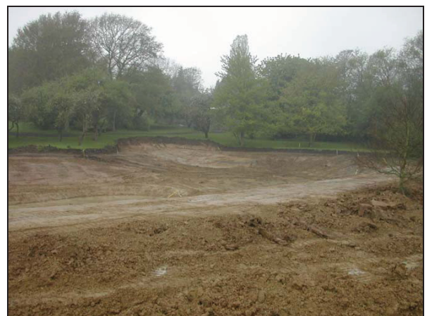
Plate 6: Excavation of lake completed, facing west-northwest
