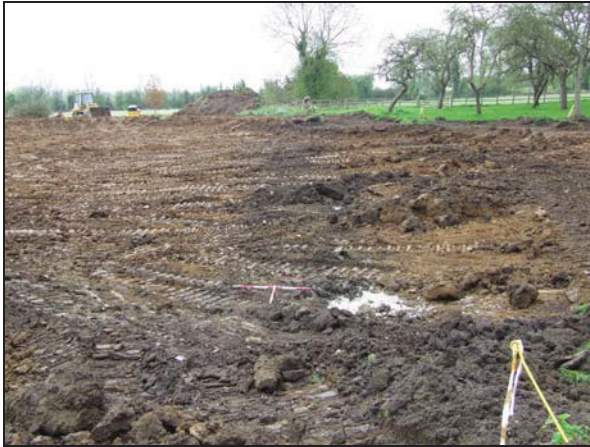
Plate 1: The ditches aligned with extant field boundary, facing south-southwest
