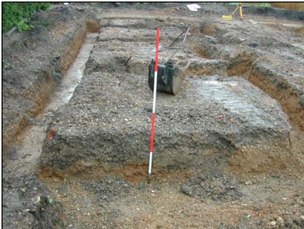
Plate 3: Foundations detail N
