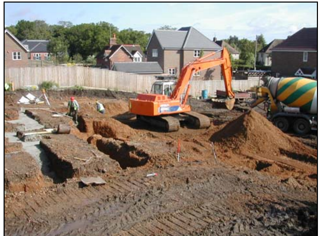
Plate 4: Foundations view N
