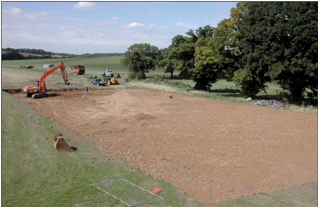
Plate 4: The site during subsoil stripping; view looking north
