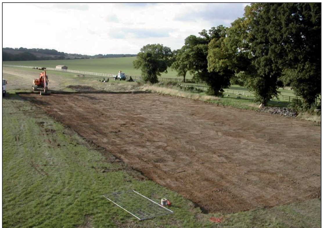
Plate 2: Completed topsoil strip; view looking north
