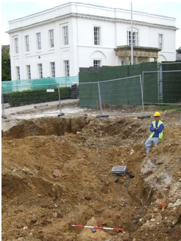
Plate 2: Culvert in foreground with Walton Hall at rear, facing NE
