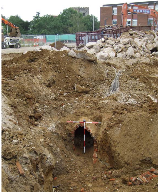
Plate 1: Culvert in foreground with Geoffrey Crowther building at rear, facing SW
