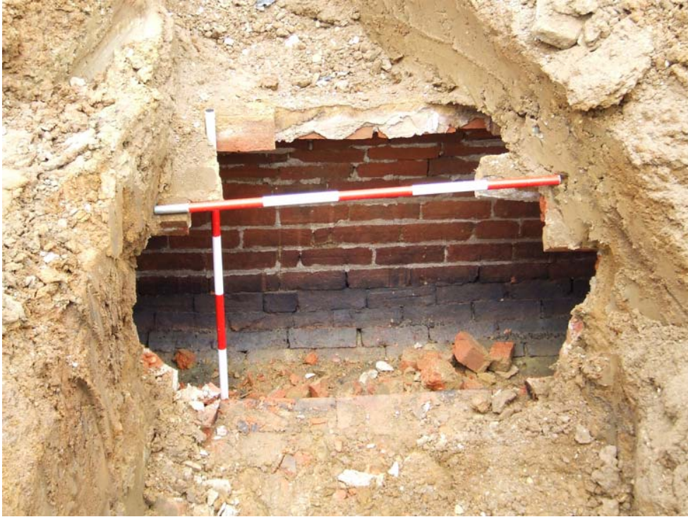
Plate 3: Southwestern part of culvert, facing NW
