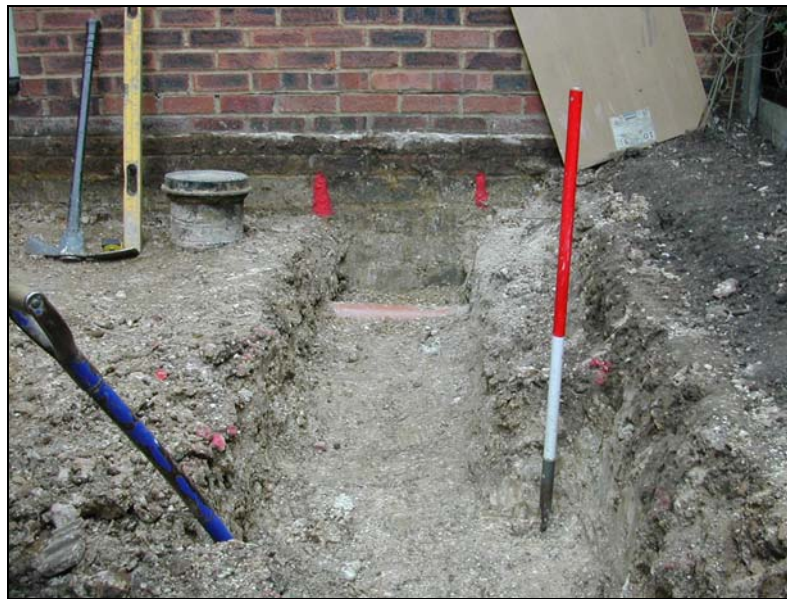
Plate 1: The building footing, after excavation ( Scale = 1m )
