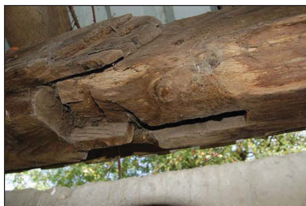
Plate 6: Scarf joint & mortice detail, northern tiebeam
