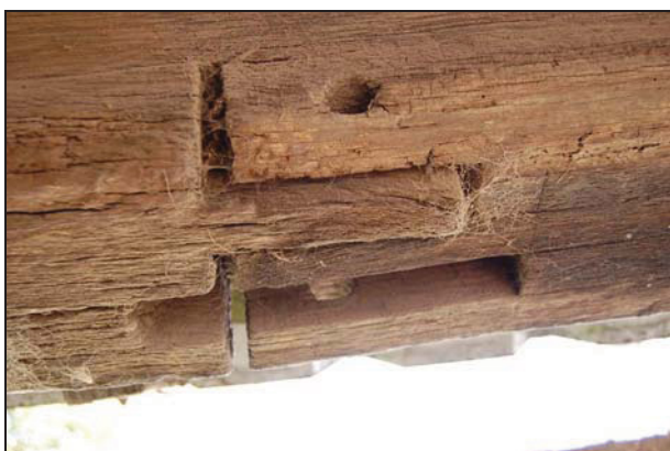
Plate 7: Scarf joint & mortice detail, east wallplate
