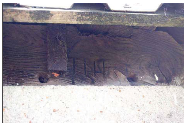
Plate 8: Carpenters assembly mark, east wallplate
