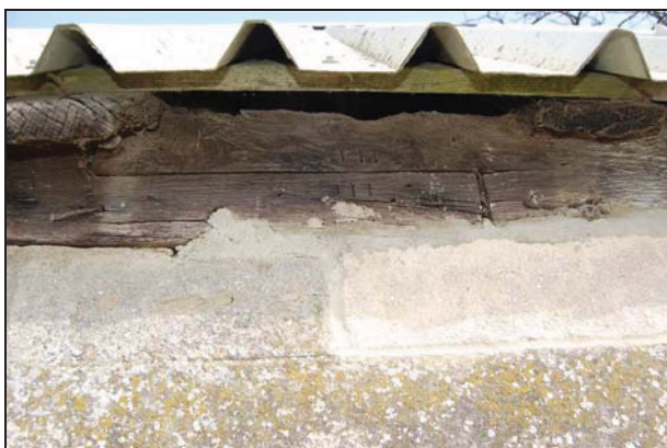
Plate 9: Scarf joint & carpenters assembly marks, west wallplate
