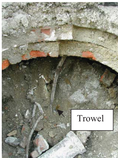
Plate 5: Detail of brick work, iron water pipe looking west
