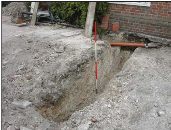
Plate 3: Detail of foundation trench looking north east
