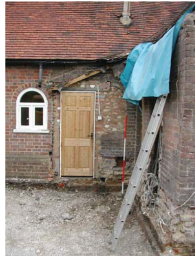
Plate 2: View east showing detail of blocked window
