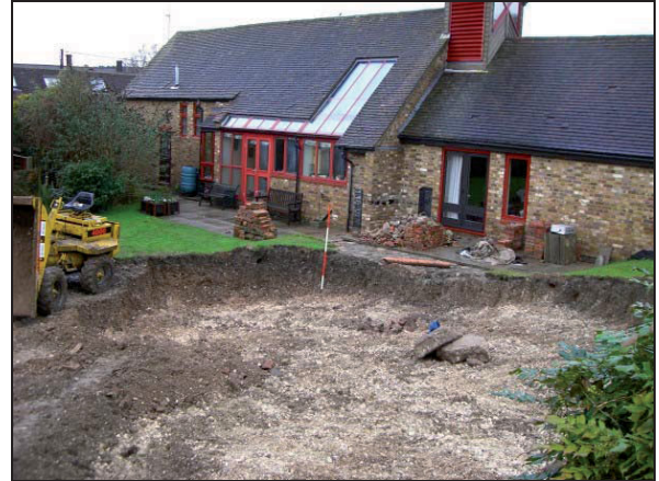
Plate 2: The site looking north west
