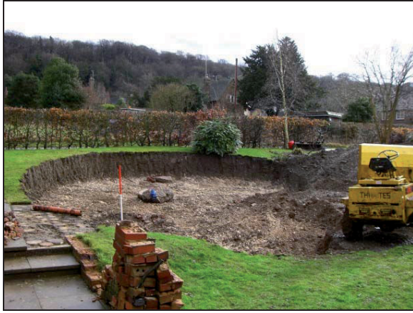
Plate 1: The site looking south east
