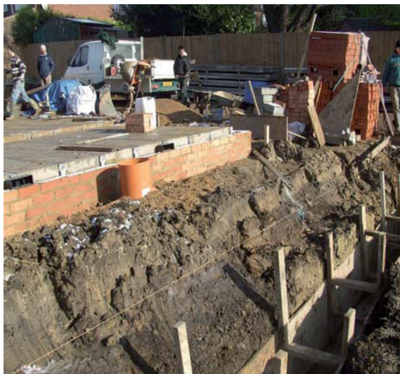
Plate 4: Completed Plot 2 footings and excavated Plot 3 trenches looking SE
