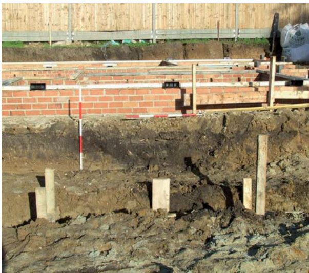
Plate 3: View of probable modern ditch in Plot 2 footings, looking NNE
