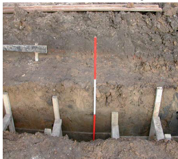
Plate 6: Section of Plot 4 footing trenches
