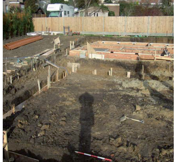
Plate 2: Footings of Plots 1 and 2 looking NNW
