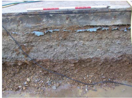
Plate 4: Section in eastern footing trench, facing SE
