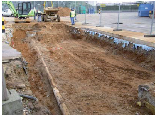
Plate 2: Western footing trench, facing NE
