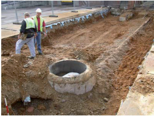
Plate 1: Western footing trench, facing S
