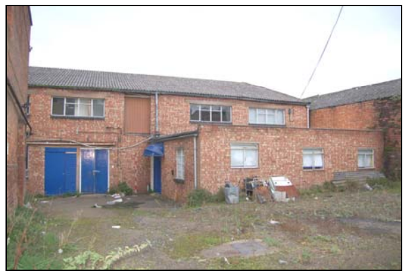
Plate 36: Canalside range: north end, looking west
