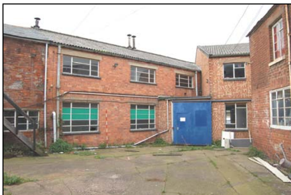
Plate 35: Canalside range: south end, looking west
