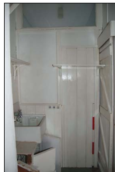
Plate 22: 50-52: F4, looking west
