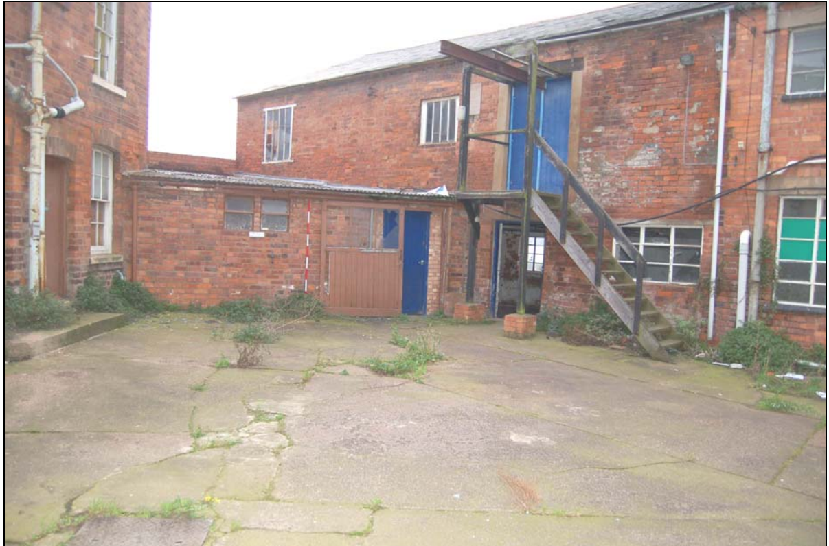
Plate 27: Warehouse and link building, looking south
