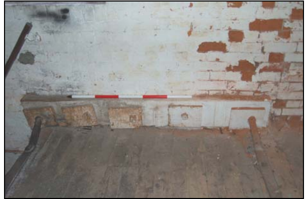
Plate 33: Warehouse: first floor, detail of crane mountings
