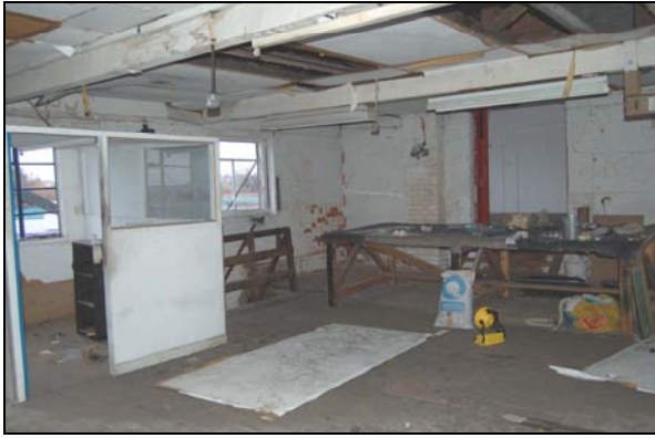
Plate 32: Warehouse: first floor, looking north-west
