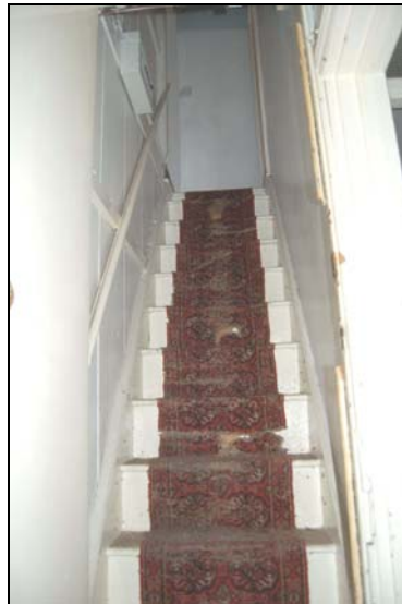
Plate 25: 52: stairs, looking south
