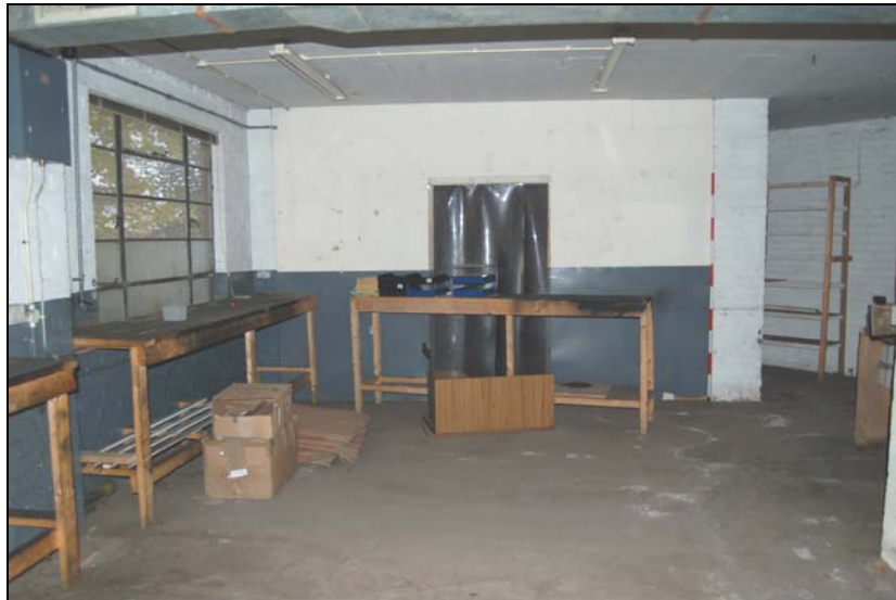
Plate 38: Canalside range: ground floor, south end, looking north-west
