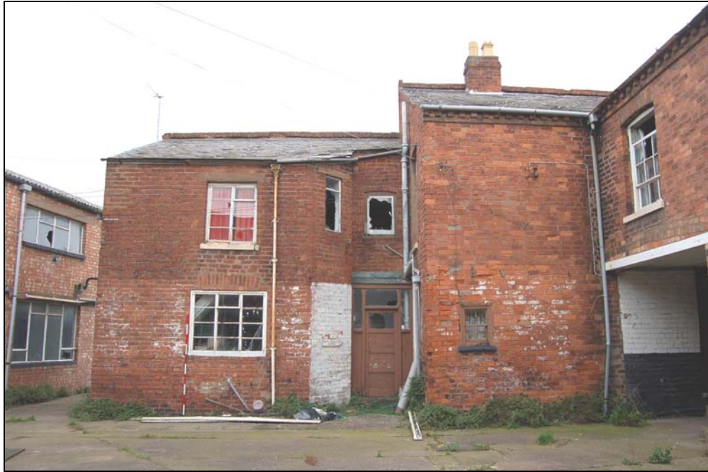
Plate 7: 48: south elevation, looking north
