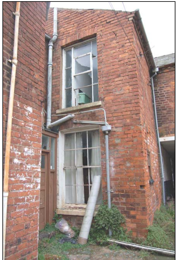
Plate 6: 48: west elevation of main building, looking east
