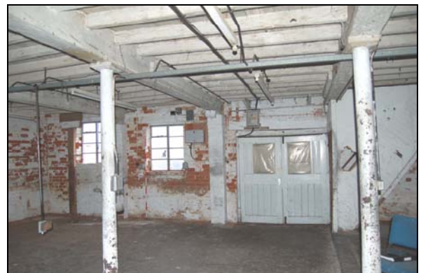
Plate 29: Warehouse: ground floor, looking west
