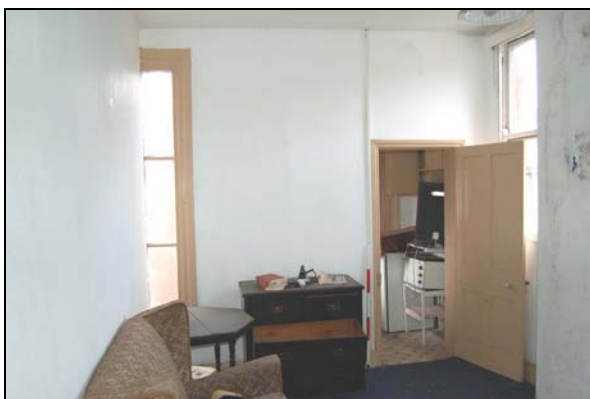
Plate 16: 48: F7, looking west
