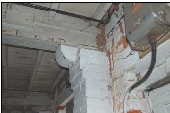
Plate 30: Warehouse: ground floor, corbel and supporting pier on west wall
