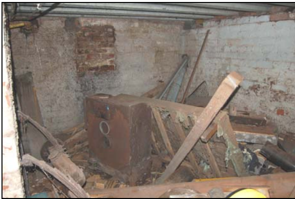
Plate 8: 48: cellar, looking south-east
