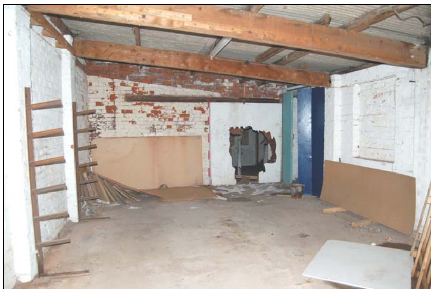
Plate 39: Link building: interior, looking west
