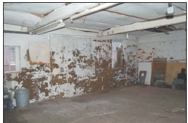
Plate 31: Warehouse: first floor, looking south
