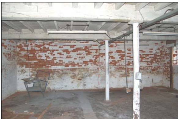
Plate 28: Warehouse: ground floor, looking south
