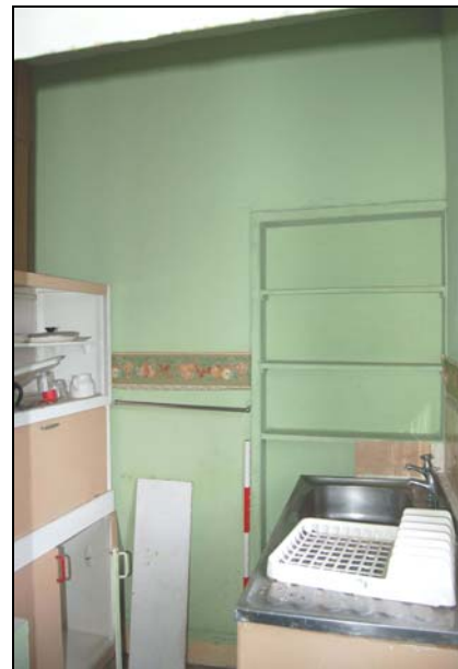
Plate 15: 48: F5, looking west
