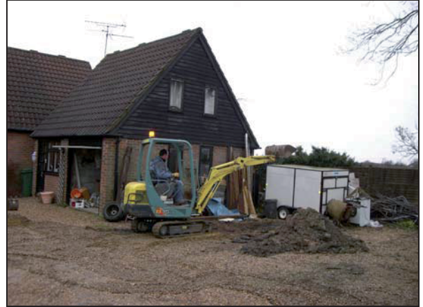
Plate 2: Evaluation trenching in progress
