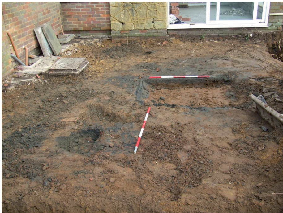
Plate 2: Shallow modern features revealed by removal of patio, facing NE
