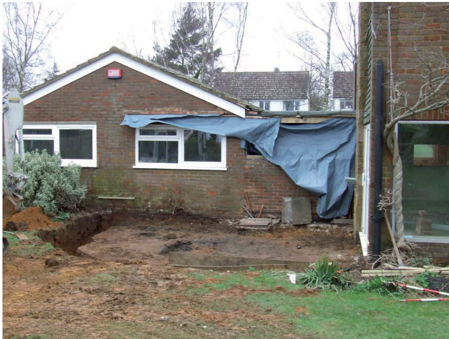
Plate 4: Groundwork completed, facing NNW
