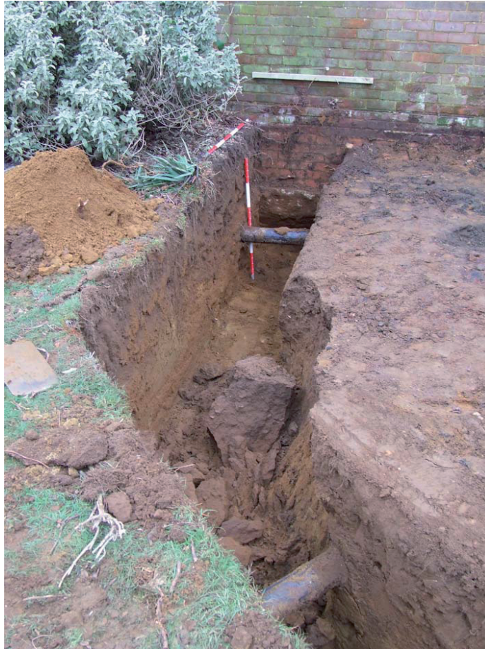
Plate 3: Foundation trench, facing NW
