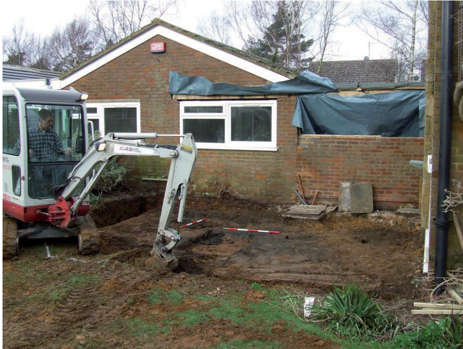
Plate 1: Excavation of foundation trenches, facing NW
