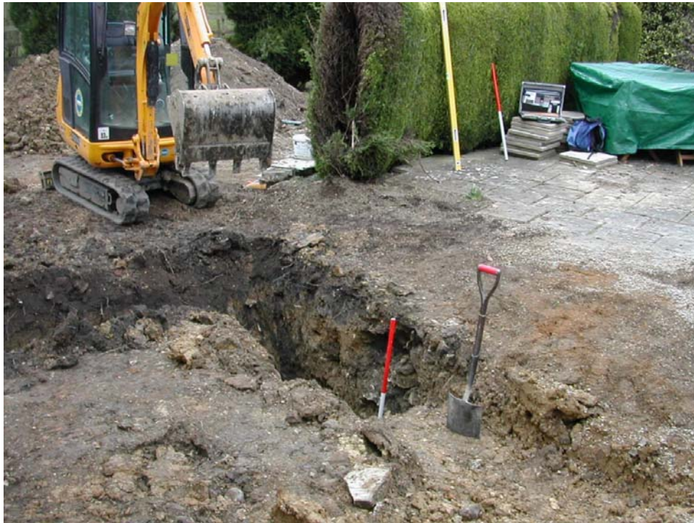
Plate 3: General view of location of feature (scale = 1m)
