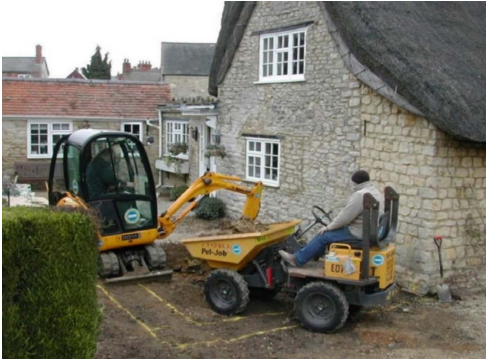
Plate 1: General working view
