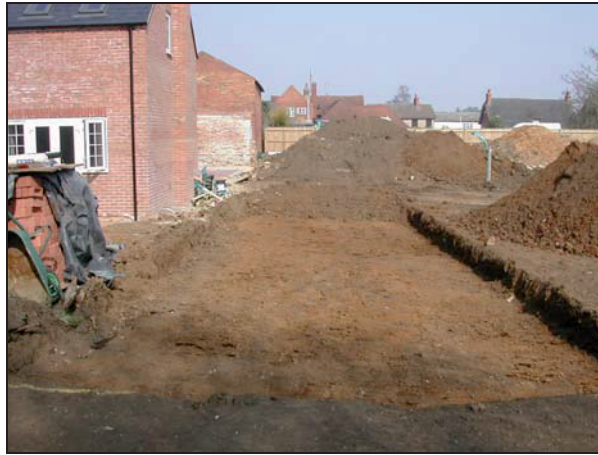
Plate 1: View east across part of the new access road
