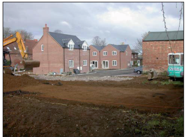
Plate 4: Looking north with the ground reduction underway
