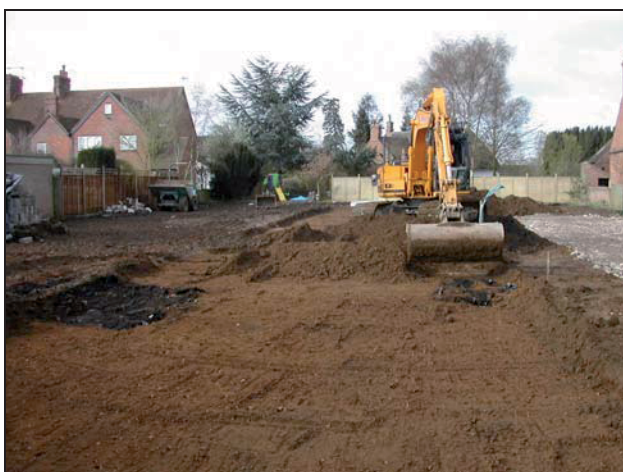
Plate 5: Looking west with ground reduction in progress
