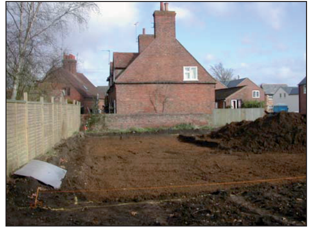
Plate 2: Western end of the site after ground reduction
