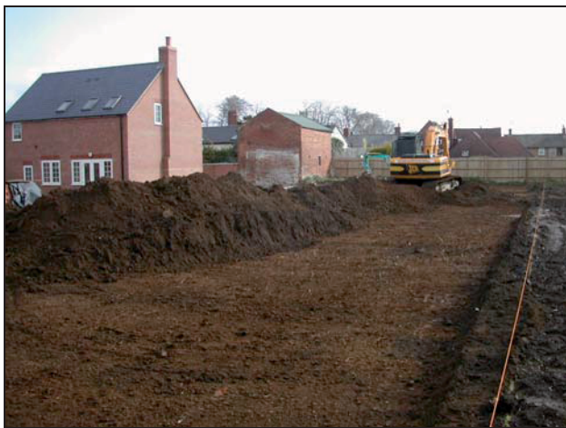
Plate 3: View east across reduced level
