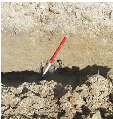
Plate 5: Well or Soakaway [2] partially revealed in northern footing of house.
