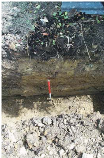
Plate 3: Section of eastern house footing, topsoil and natural subsoil are visible.
