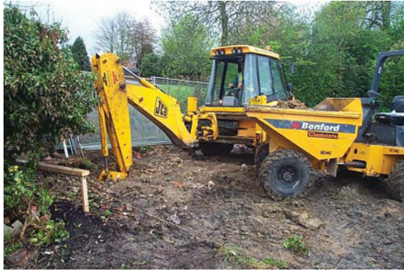
Plate 1: Southern footings of house under excavation.
