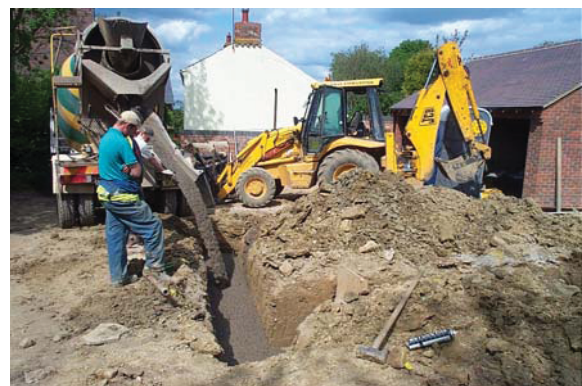
Plate 6: House footings during concrete pouring.
