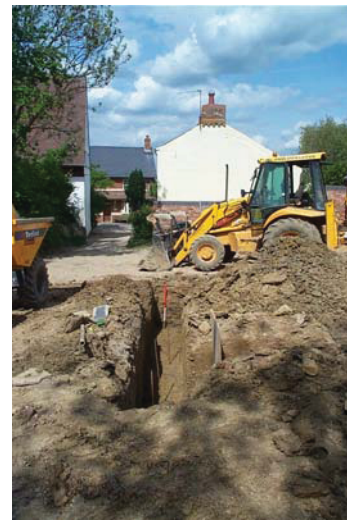
Plate 4: Western footings of house.
