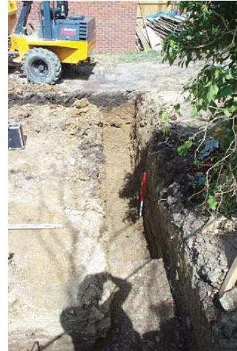
Plate 2: Eastern footings of house under excavation.
