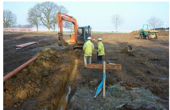
Plate 4: Service trenches in the south of the site. Facing north.
