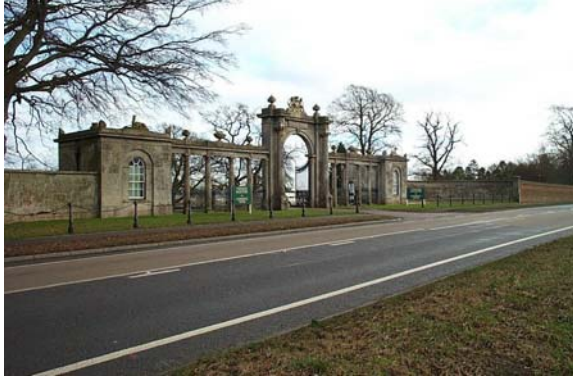
Plate 1: Now the entrance to Towcester Racecourse, and the development area, the 'Chain Gate' was originally built in 1824. This was the entrance to Easton Neston Park.
