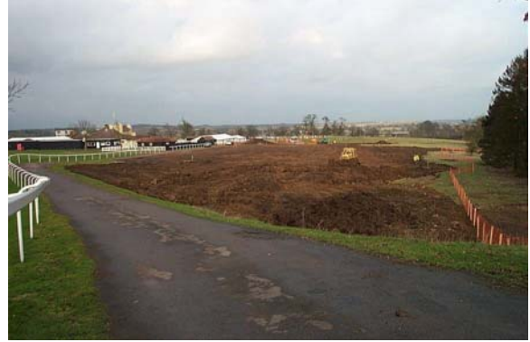
Plate 2: Work in progress, view from Watling Street.
