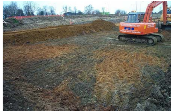
Plate 2: Stripping on the main roundabout, piers 1 – 4.
