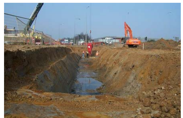
Plate 6: Natural subsoil visible in culvert sections, facing west.
