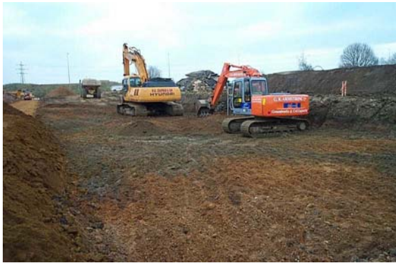
Plate 1: Stripping on the main roundabout, piers 1 – 4.
