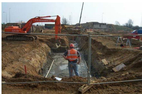
Plate 5: Culvert during excavation, facing east.
