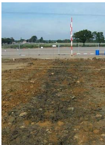
Plate 5: Base of tarmac access road after removal, facing north
