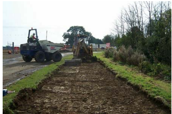
Plate 4: Topsoil stripping on the service run, northwest of main Development Area.
