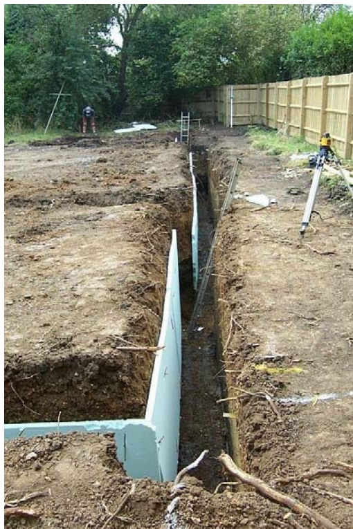
Plate 4: Excavation of house footings
