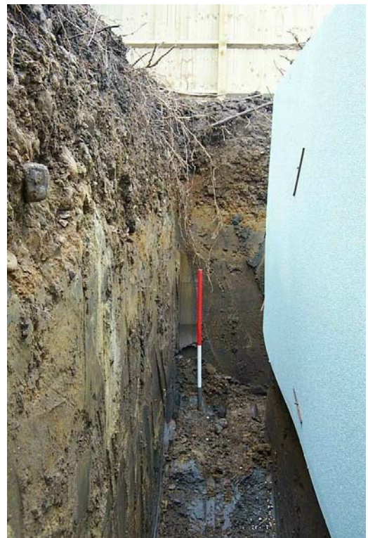
Plate 5: Section of house footings
