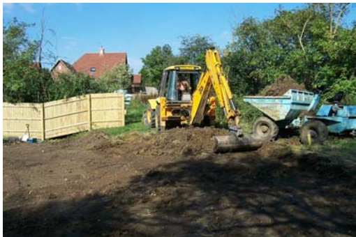
Plate 1: Topsoil Stripping House plot
