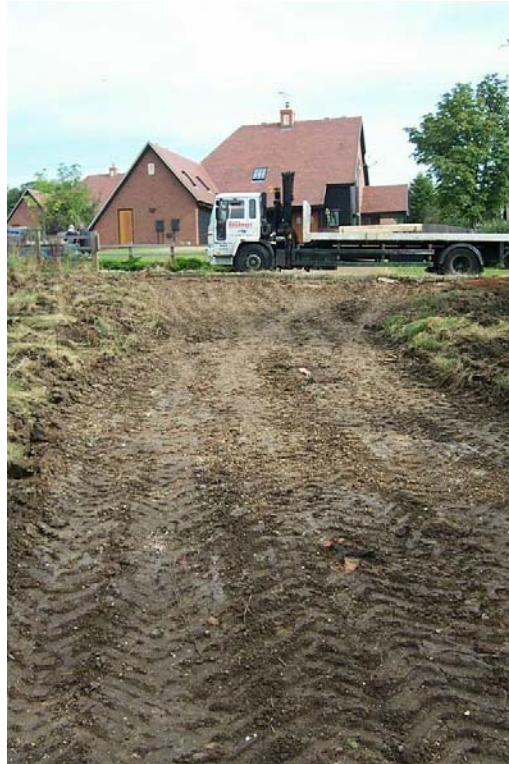
Plate 3: Topsoil Stripping Driveway
