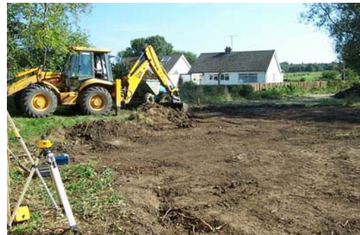
Plate 2: Topsoil Stripping House plot
