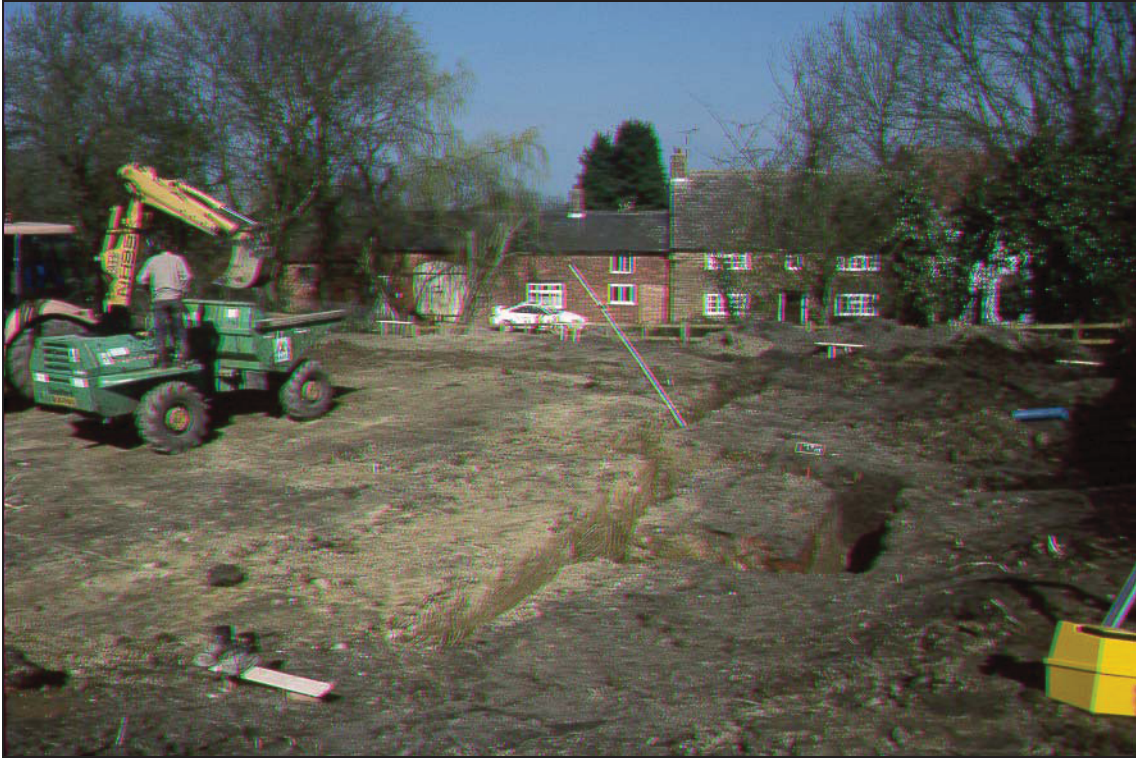
Plate 5: House footings during excavation
