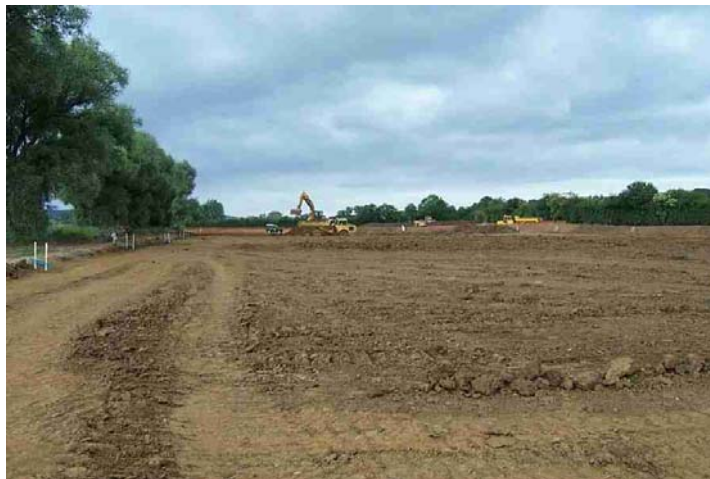
Plate 10: Borrow pit during topsoil stripping
