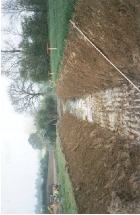
Plate 3: Excavation of river diversion through alluvium and natural subsoil
