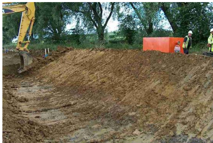
Plate 11: Excavation of Borrow pit through alluvium
