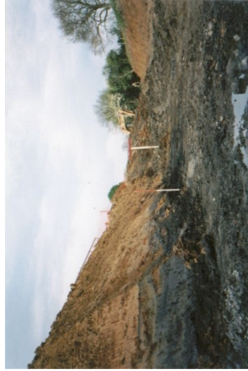
Plate 3: Excavation of river diversion through alluvium and natural subsoil
