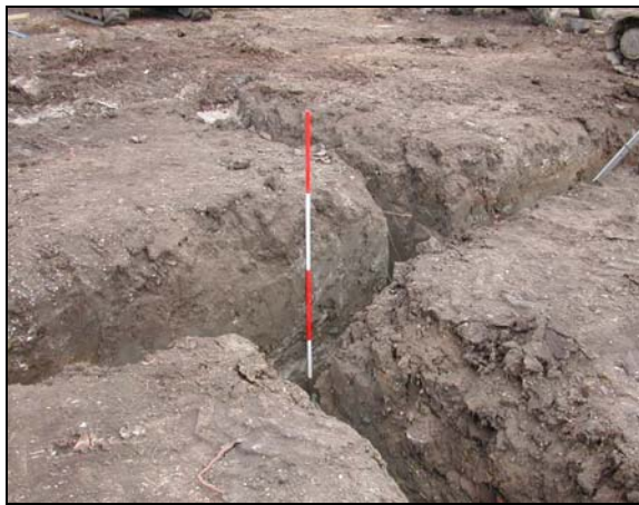
Plate 9: Plot 1 foundations looking north west
