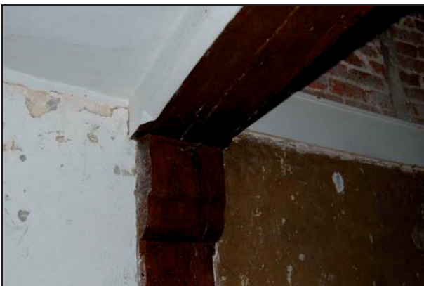
Plate 17: G1: ogee moulding in post
