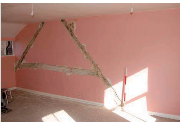
Plate 41: S3: west wall
