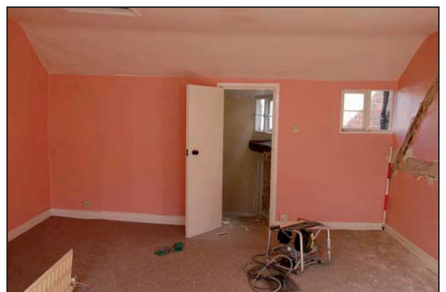
Plate 42: S3: north wall
