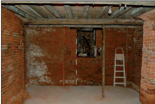
Plate 3: Cellar: C1, looking south
