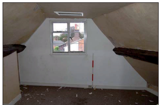
Plate 36: S2: north wall
