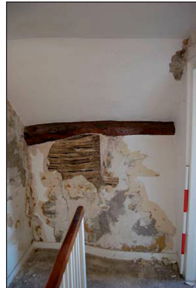
Plate 34: S1: west wall
