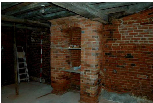
Plate 5: Cellar: C1, chimney support
