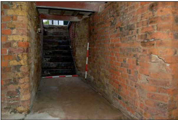
Plate 9: Cellar: entrance passage, looking north
