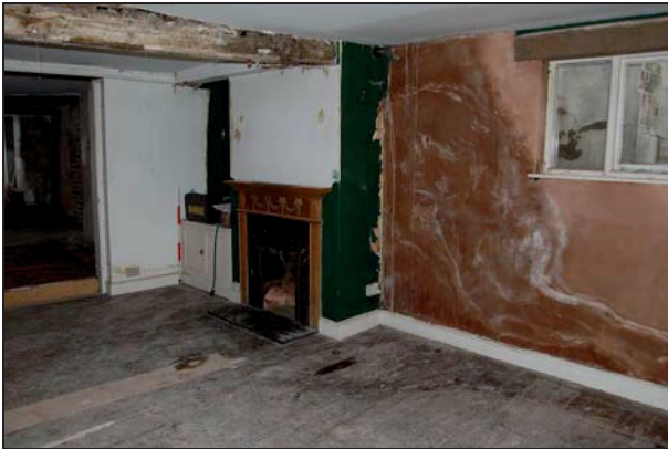
Plate 15: G1: fireplace in west wall
