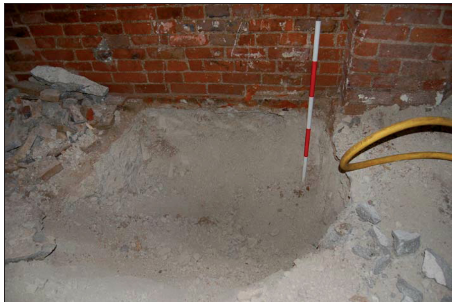
Plate 45: Underpinning pit below G1b fireplace
