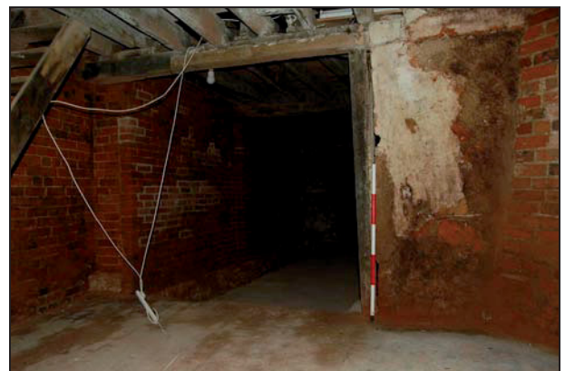
Plate 6: Cellar: C2, looking south
