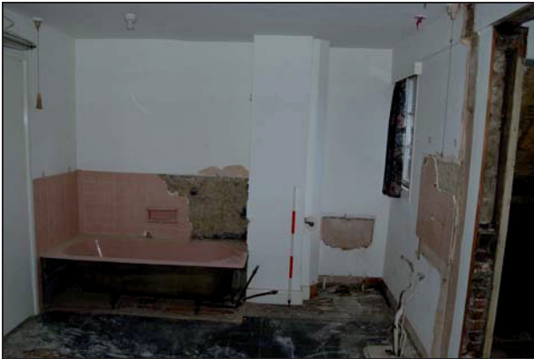
Plate 33: F3: west wall, southern end
