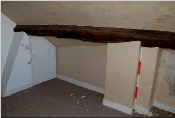
Plate 37: S2: west wall
