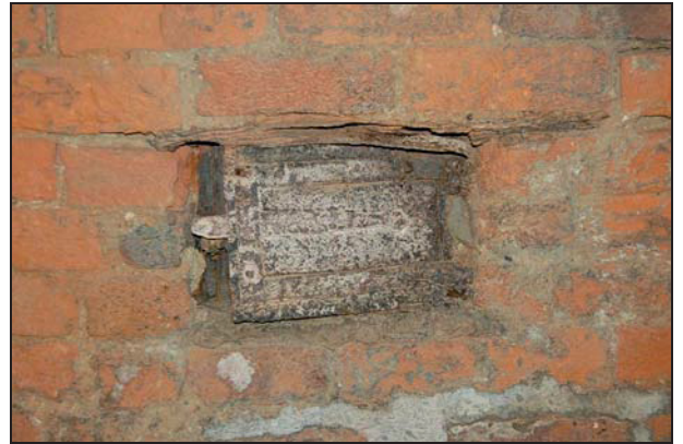
Plate 8: Cellar: C2, hatch detail
