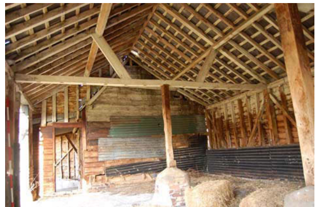
Plate 12: Barn 2: north elevation
