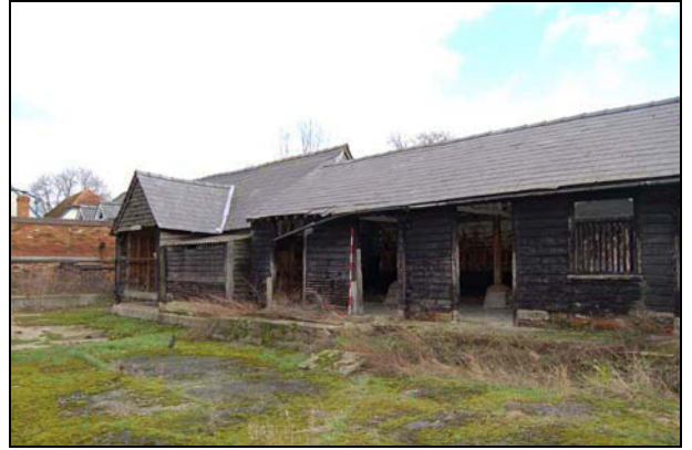
Plate 2: Barns 1-2: west elevation
