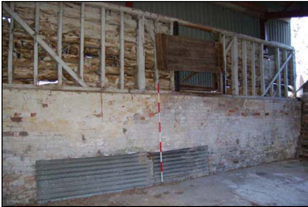
Plate 31: Barn 4: west wall, northern end
