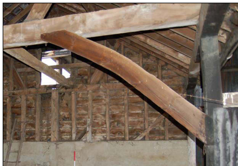
Plate 48: Barn 5 truss detail
