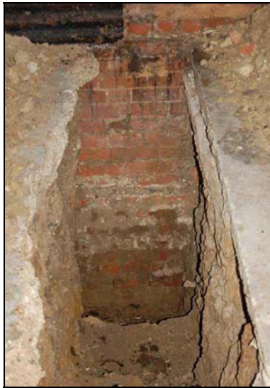
Plate 15: Barn 2: test pit in SE corner
