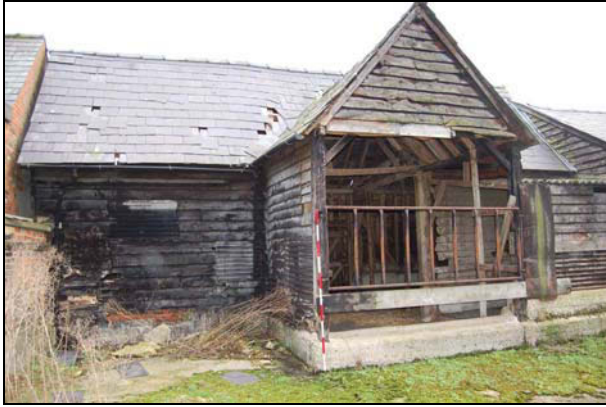
Plate 1: Barn 1: west elevation
