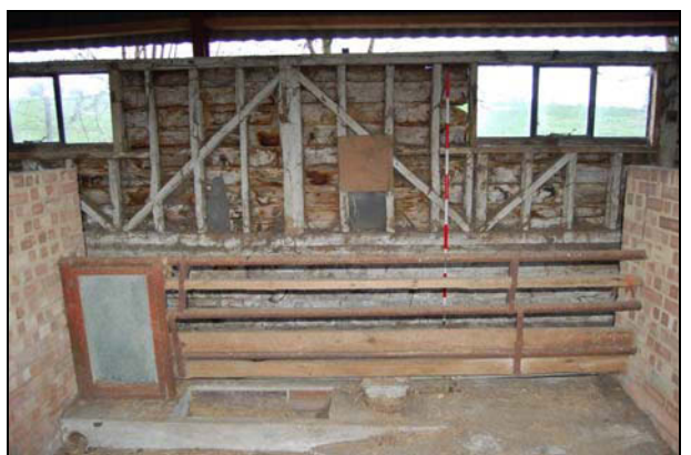
Plate 30: Barn 4: pig pen & west wall detail
