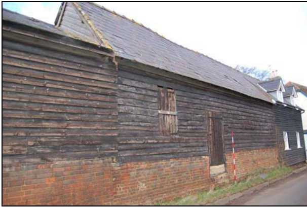
Plate 3: Barns 1: east elevation
