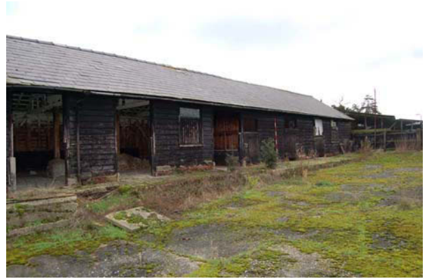
Plate 20: Barns 2 & 3: west elevation
