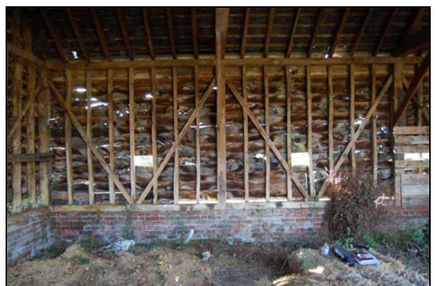
Plate 36: Barn 5: south wall detail
