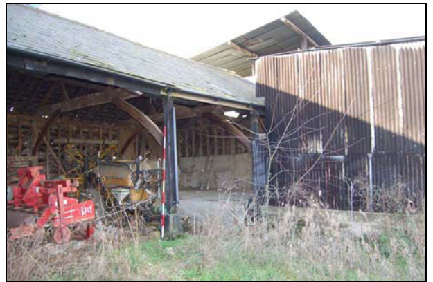
Plate 40: West end of Barn 5 & adjoining outbuilding
