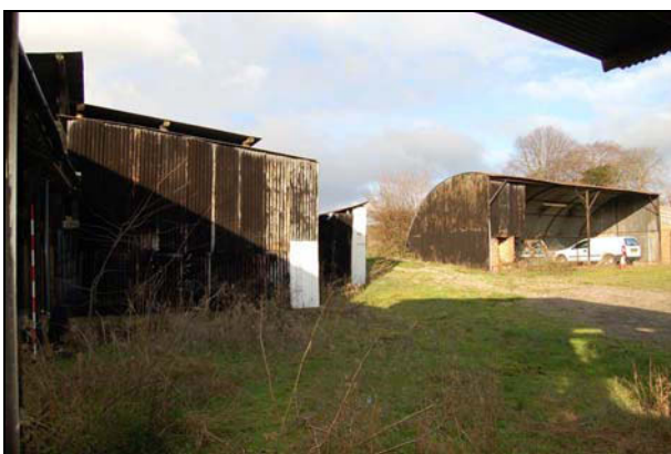
Plate 41: Outbuildings north & NW of Barn 5
