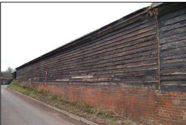
Plate 11: Barns 2 & 3: east elevation
