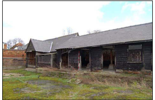
Plate 10: Barns 1 & 2: west elevation
