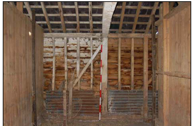
Plate 16: Barn 2: 2 nd subdivision, looking east
