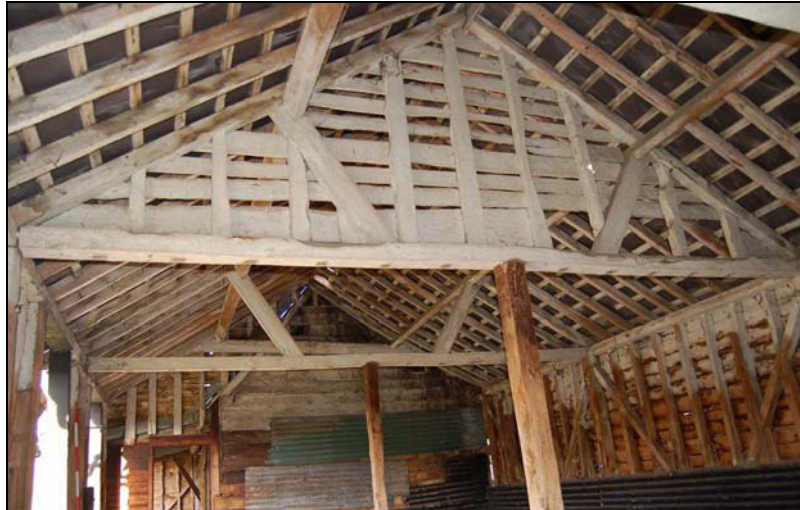
Plate 46: Barn 2 truss detail
