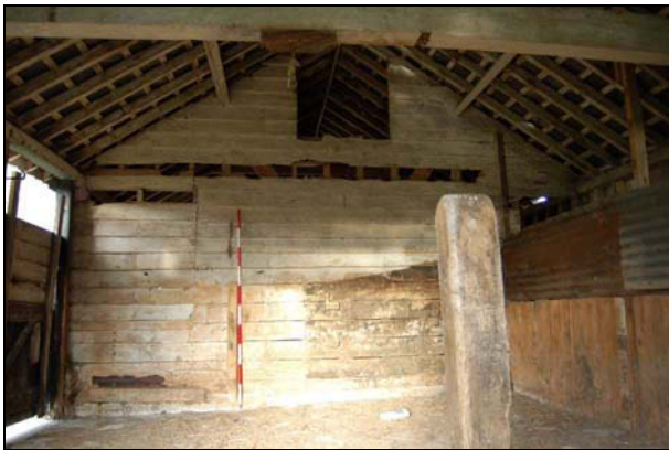
Plate 21: Barn 3: north wall
