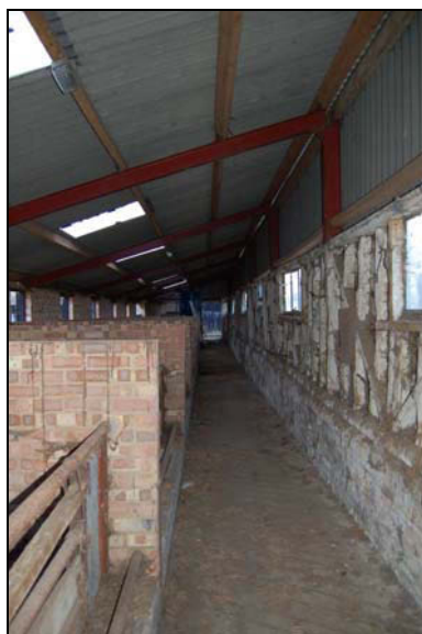
Plate 29: Barn 4: looking south
