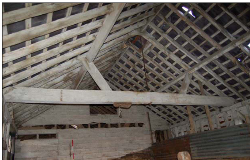
Plate 47: Barn 3 truss detail
