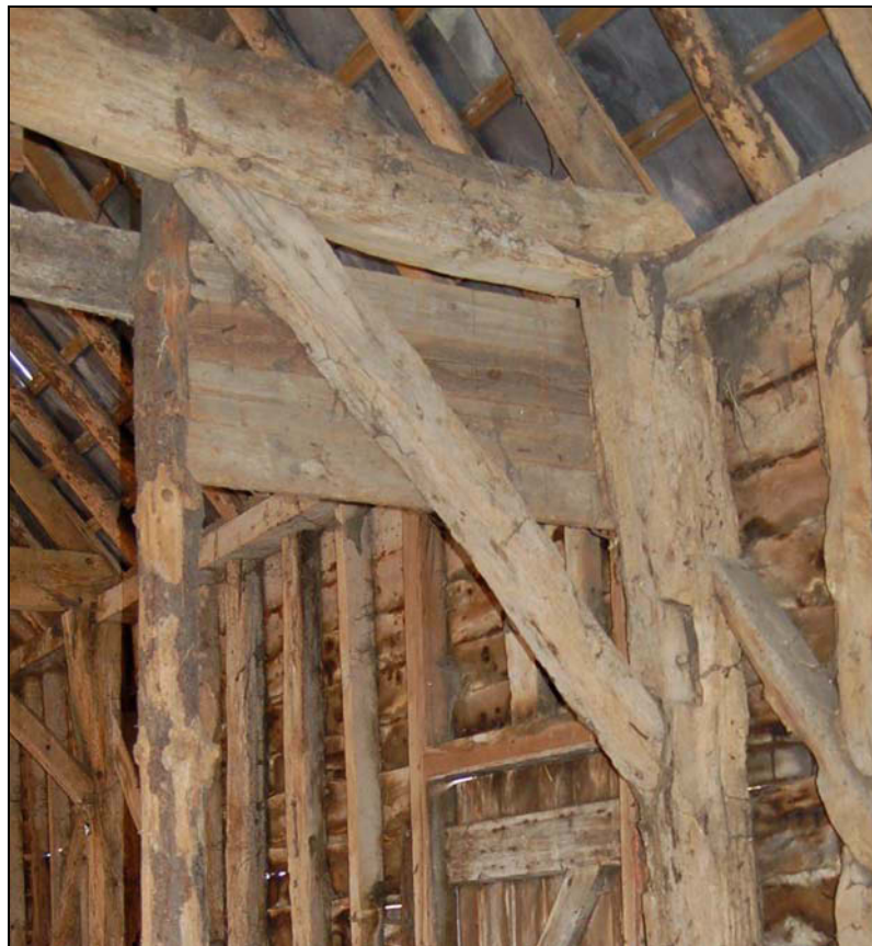
Plate 45: Barn 1 truss detail
