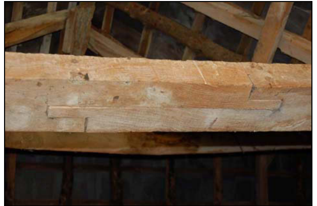
Plate 44: Face halved & counterbladed scarf joint as seen in Barn 1
