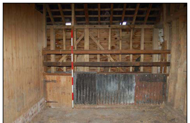
Plate 18: Barn 2: 3 rd subdivision, looking east
