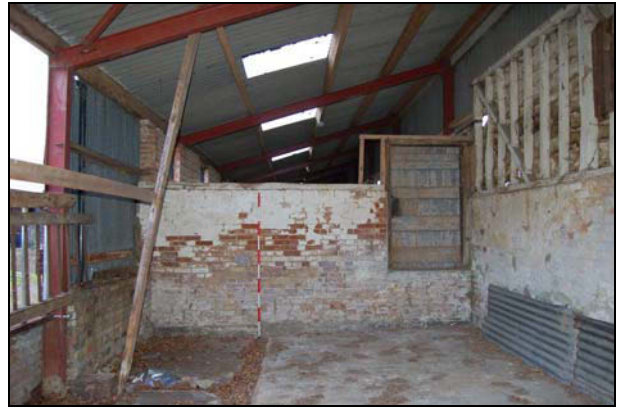
Plate 32: Barn 4: south wall of northern end
