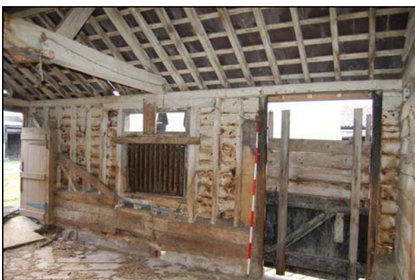
Plate 23: Barn 3: west wall
