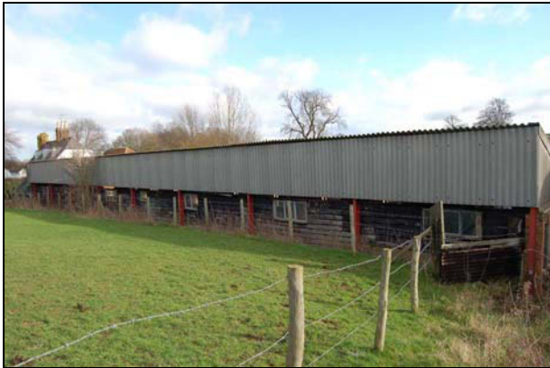
Plate 27: Barn 4: west elevation
