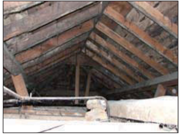
Plate 27: Roof structure above F6, looking south
