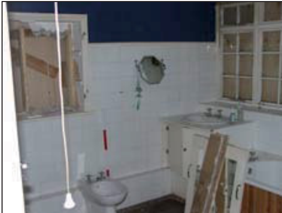
Plate 22: F6, looking north-west. Note blocked window to left
