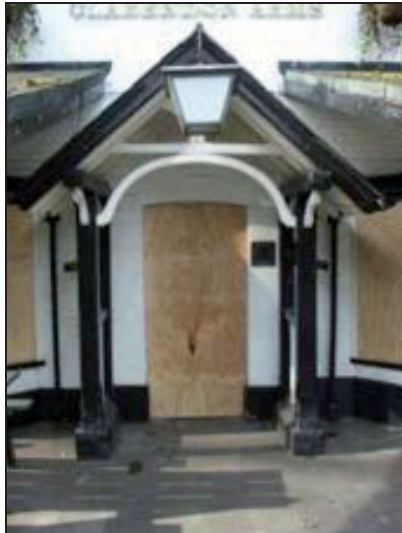
Plate 2: East elevation: porch over main entrance
