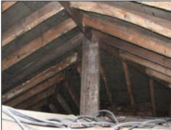
Plate 26: Roof structure above F7, looking south
