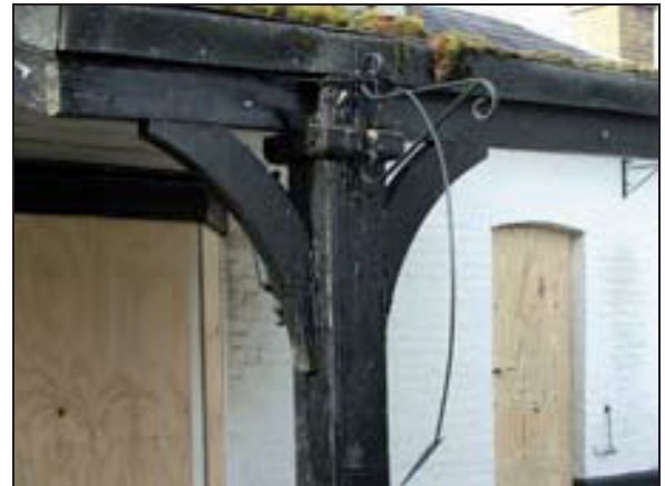
Plate 3: East elevation: detail of canopy support
