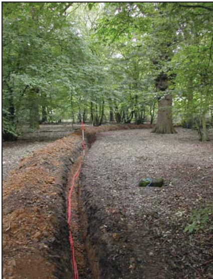
Plate 3: View looking south along cable trench
