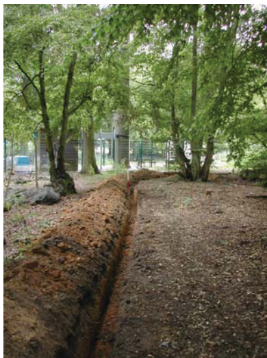
Plate 5: Cable trench near base of communications mast
