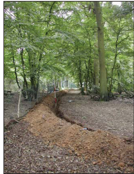
Plate 4: Further along cable trench view south
