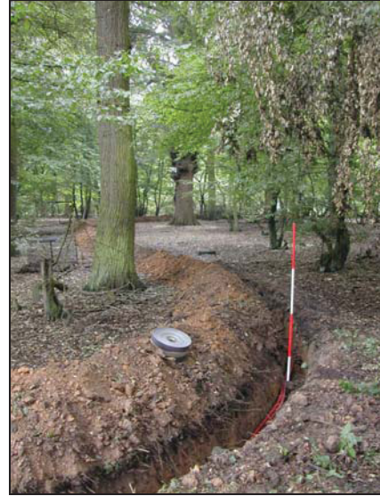
Plate 2: View looking south along cable trench
