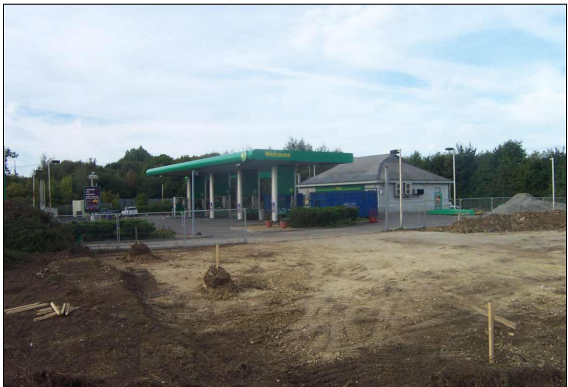
Plate 3: View showing the site in relation to the existing buildings
