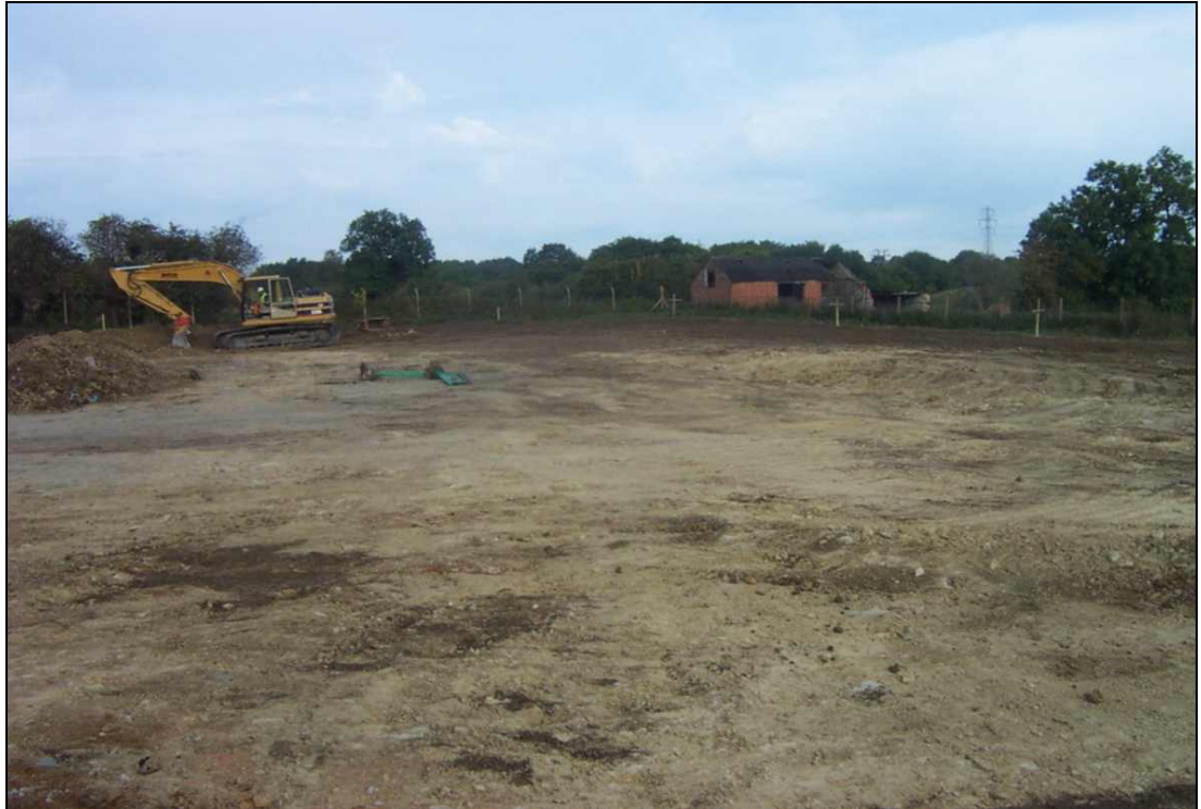
Plate 2: General view of the site during the stripping operations
