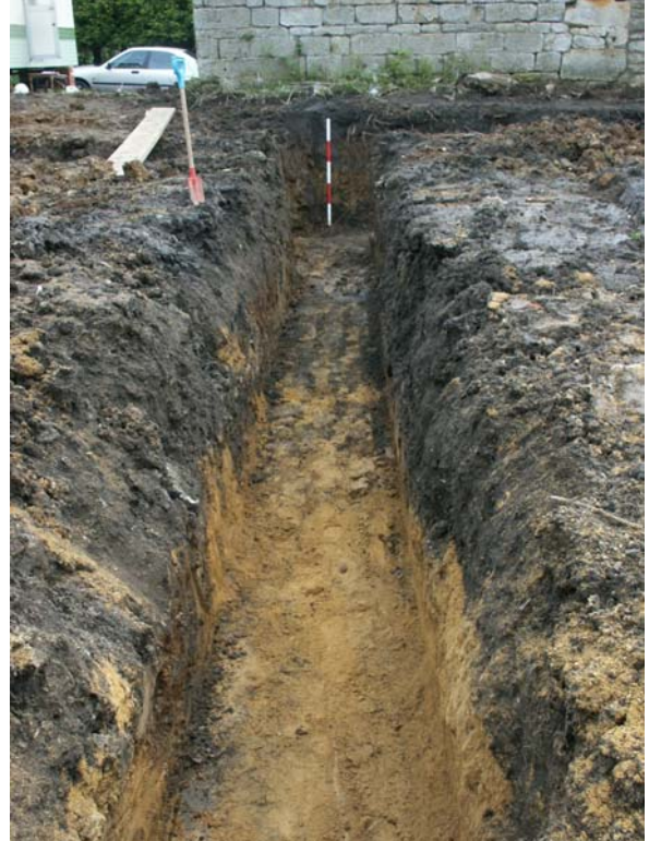
Plate 2: Footing trench looking E
