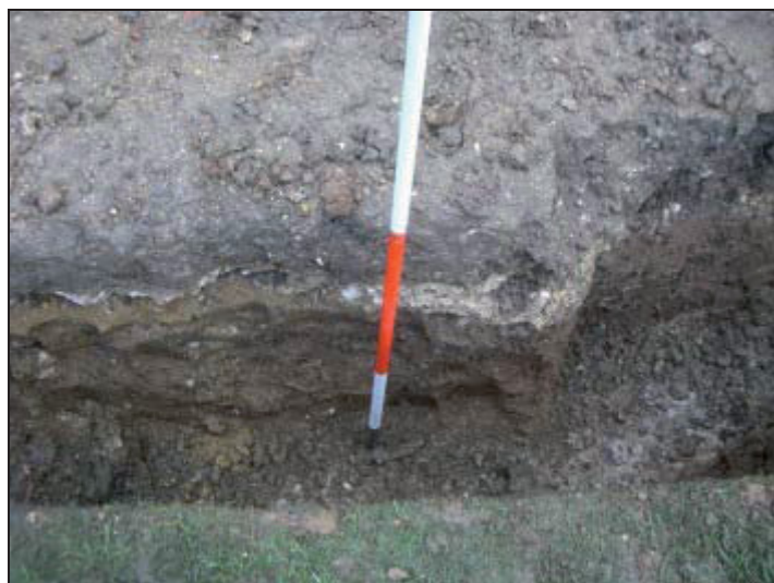
Plate 2: Detail of ground on east side of foundations
