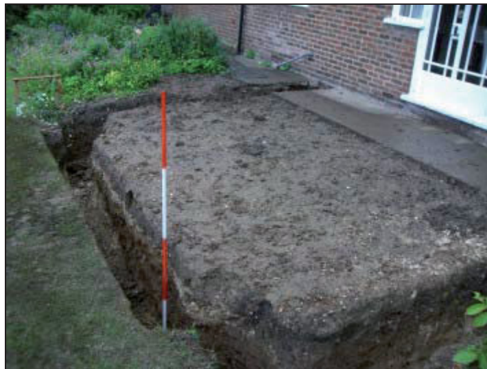
Plate 1: Oblique overall view of the foundations for the conservatory
