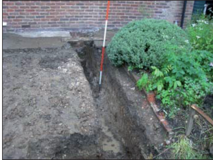
Plate 3: View of foundations on north side
