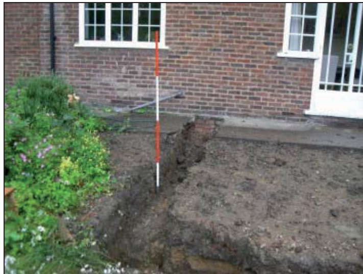
Plate 4: View of foundations on south side of conservatory
