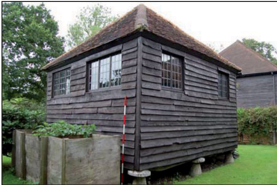
Plate 3: South & east elevations
