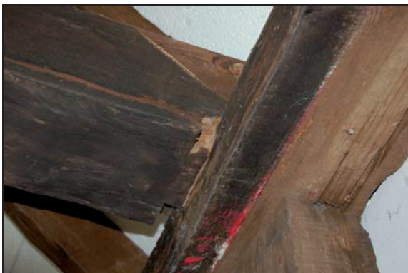
Plate 11: Tie beam joint
