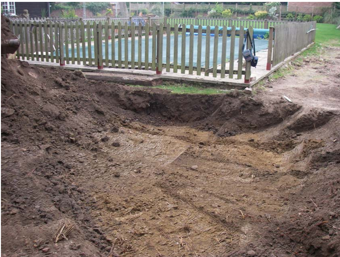
Plate 2: Typical depth of overburden removed on to the natural subsoil
