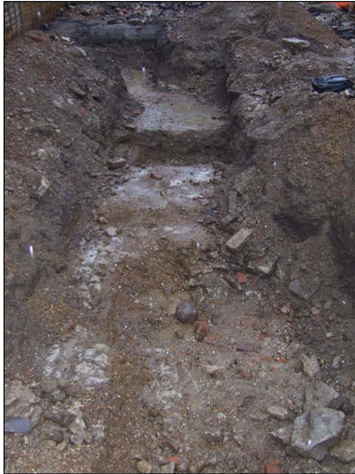
Plate 3: Trench 2, looking north east
