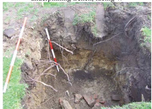
Plate 12: Section: Soakaway, facing S
