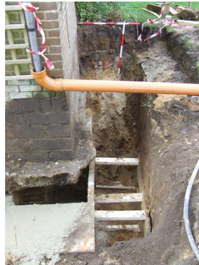
Plate 10: Brick foundation (under scale) in underpinning trench, facing W
