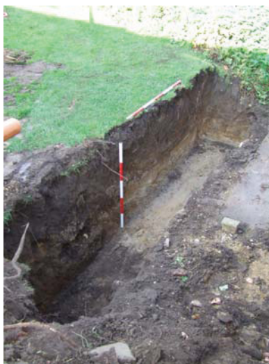
Plate 11: Footing of N – S retaining wall, facing NNE
