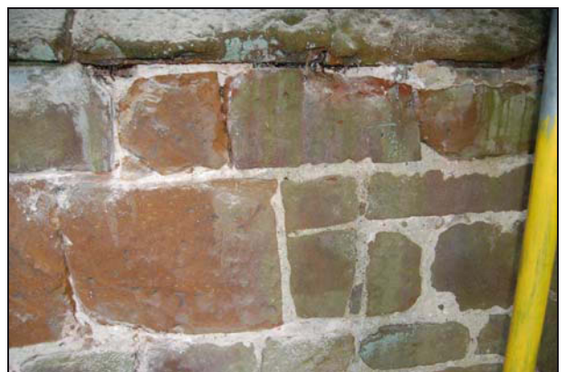
Plate 6: South elevation: Lift 1 east putlog
