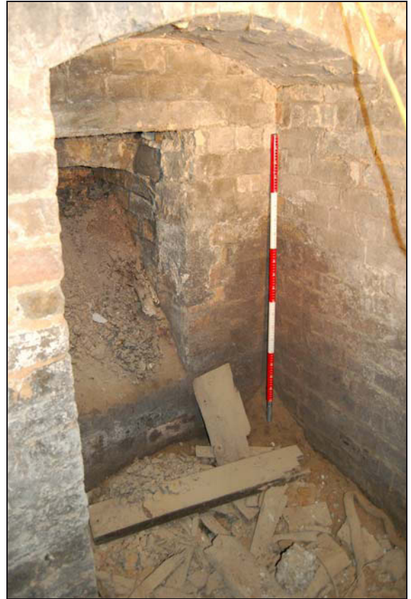
Plate 25: Cellar: looking southeast
