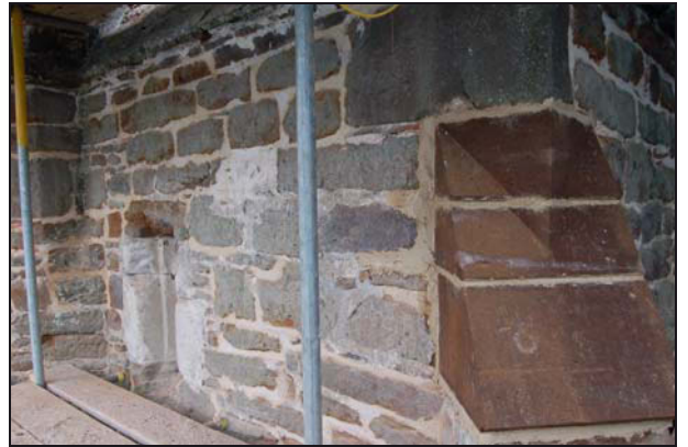
Plate 21: North buttress restoration
