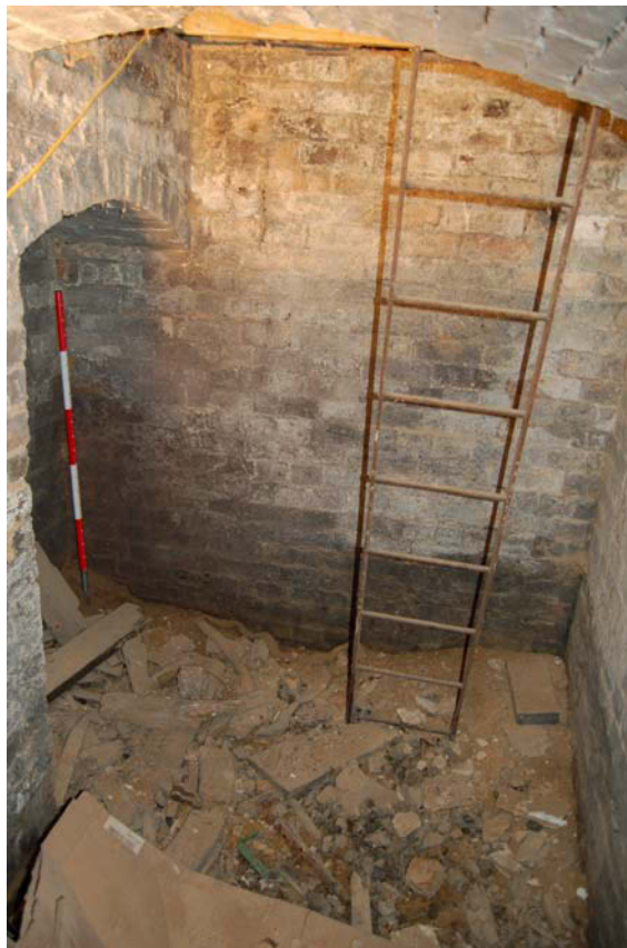
Plate 26: Cellar: looking south
