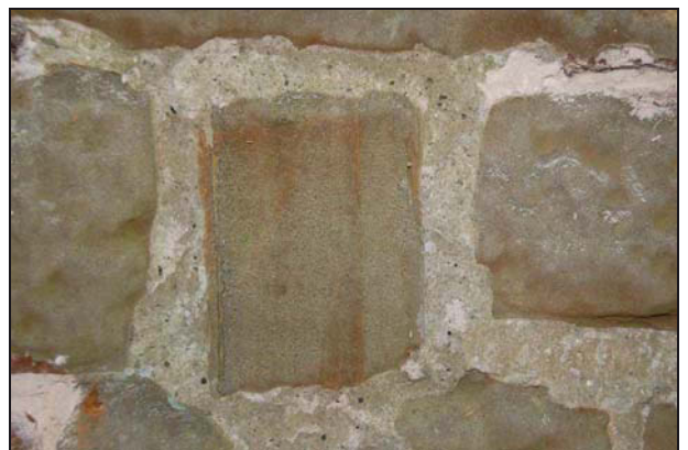
Plate 15: West elevation: Lift 2, south putlog hole
