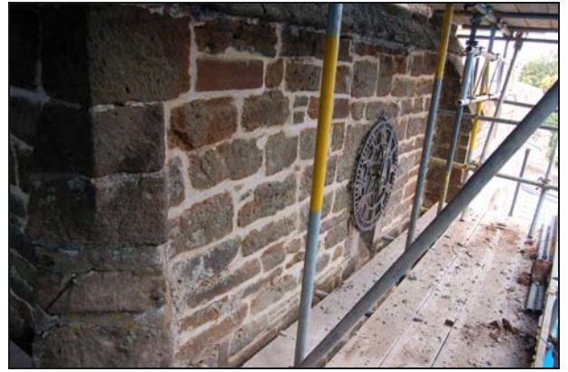
Plate 8: South elevation: clock area after restoration
