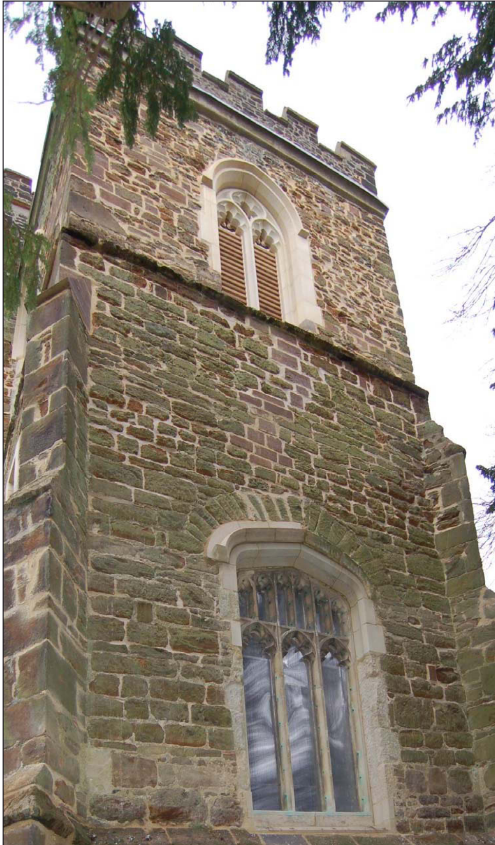
Plate 18: Upper stages of the west elevation after restoration
