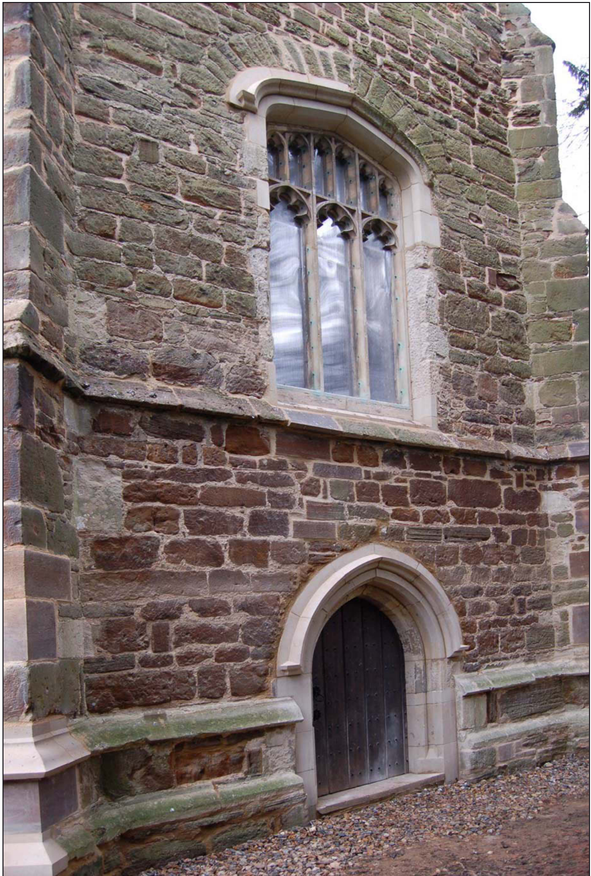
Plate 19: Lower stages of the west elevation after restoration
