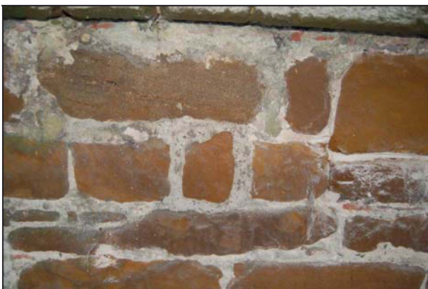
Plate 14: West elevation: Lift 1, north putlog hole
