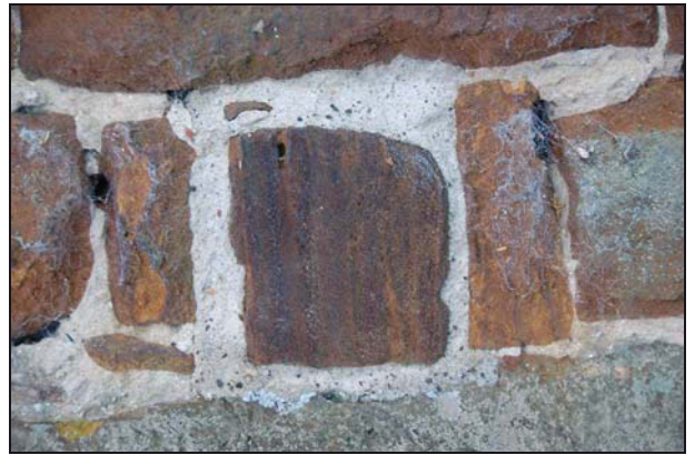
Plate 17: West elevation: Lift 4, north putlog hole
