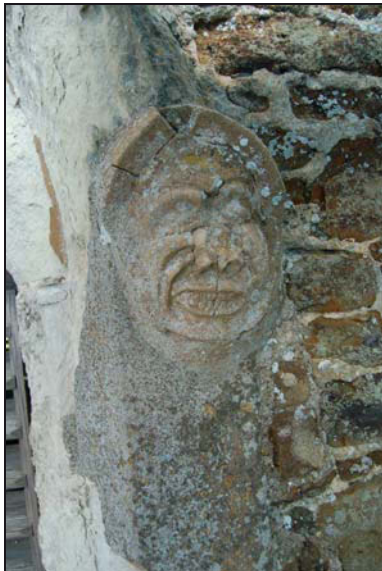
Plate 12: West elevation: belfry label stop
