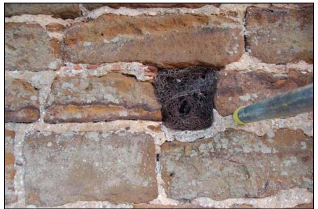
Plate 4: South elevation: Lift 4 east putlog
