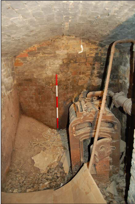
Plate 24: Cellar: looking north
