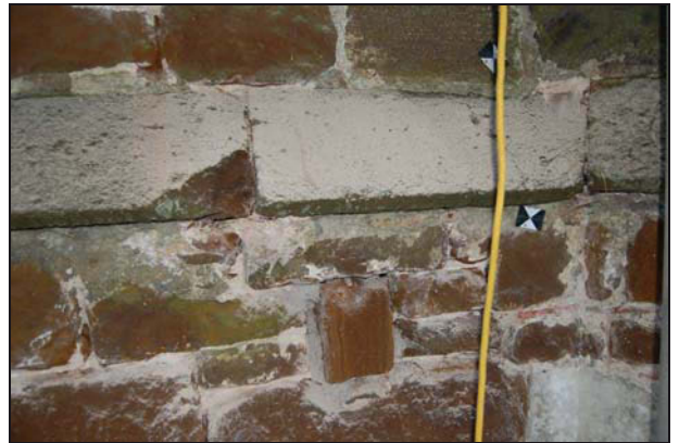
Plate 13: West elevation: Lift 1, south putlog hole
