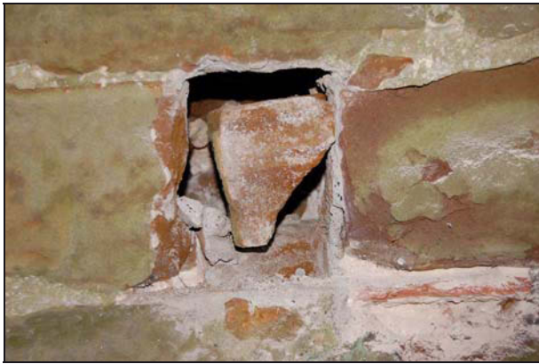
Plate 16: West elevation: Lift 2, north putlog hole
