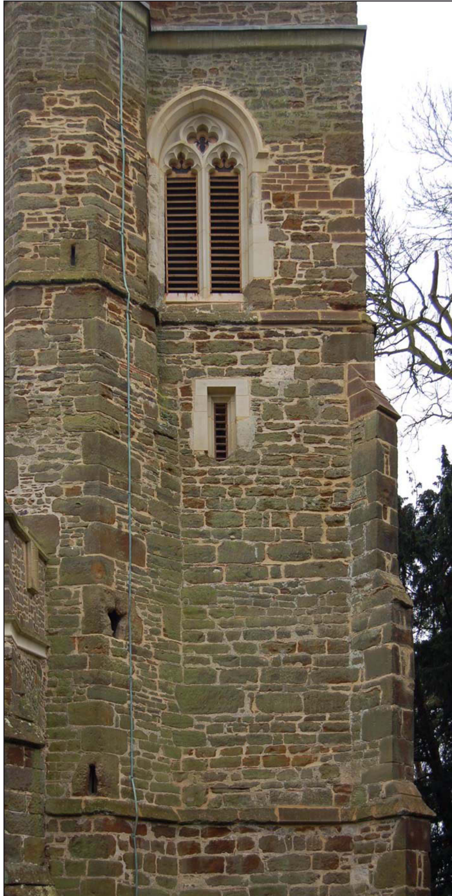
Plate 23: North elevation after restoration
