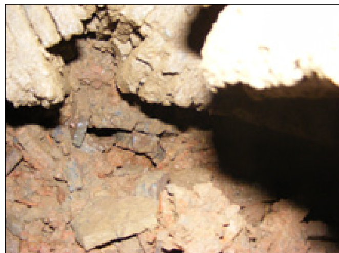
Plate 3: View inside the firing chamber, looking north beneath flue arches, showing backfill collapse
