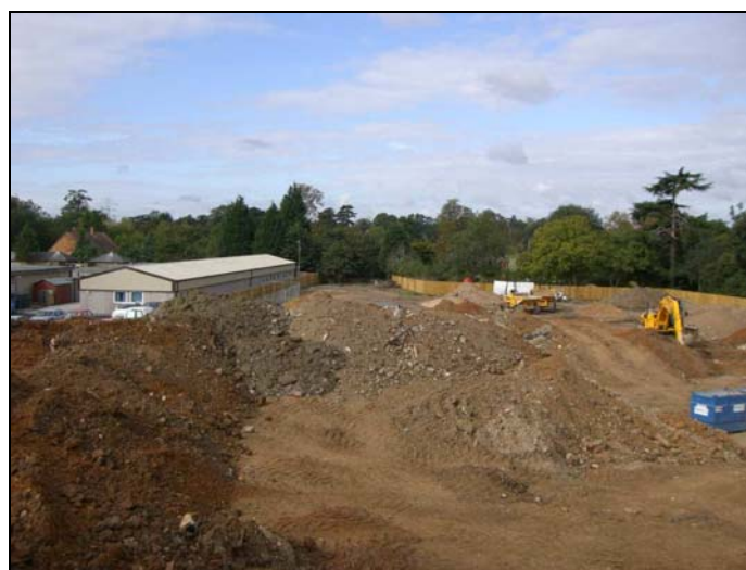
Plate 3: View looking west showing large spoil heap
