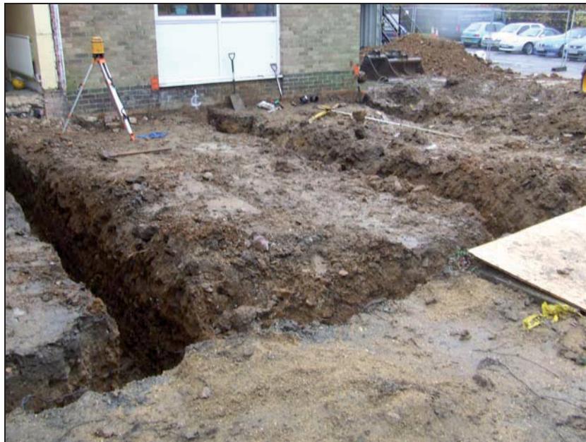
Plate 4: Overview of footings trenches
