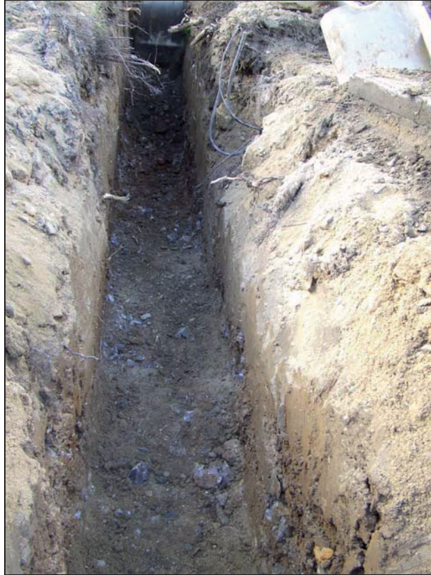
Plate 1: Service trench showing layer of sand below concrete paving
