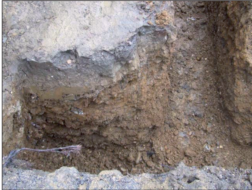
Plate 3: Section of footings trench
