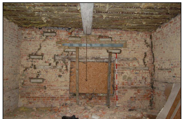
Plate 18: Room G1: west wall
