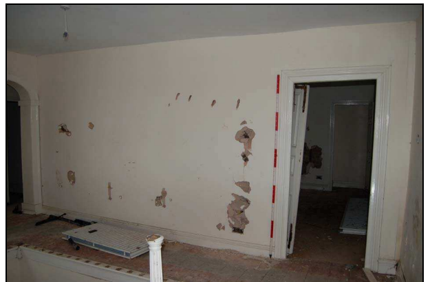
Plate 46: Room F1: east wall
