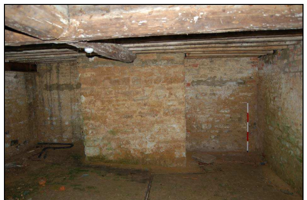
Plate 12: Cellar C2: west wall
