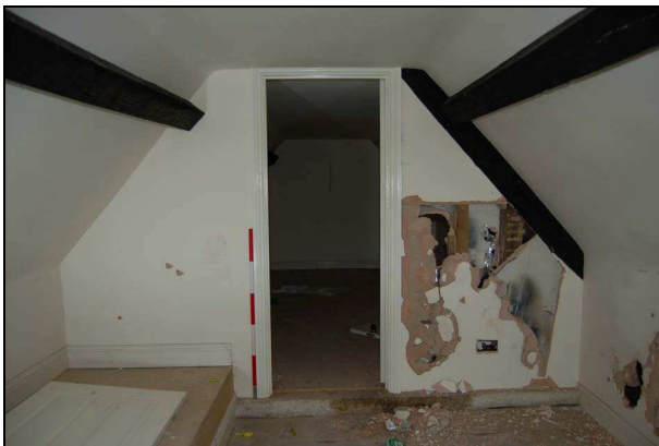
Plate 63: Room S2: west wall
