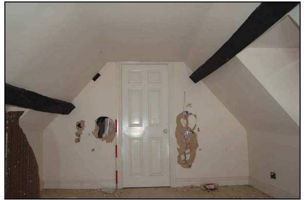
Plate 68: Room S3: east wall
