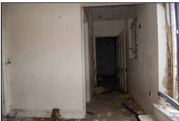
Plate 41: Room G6: looking north
