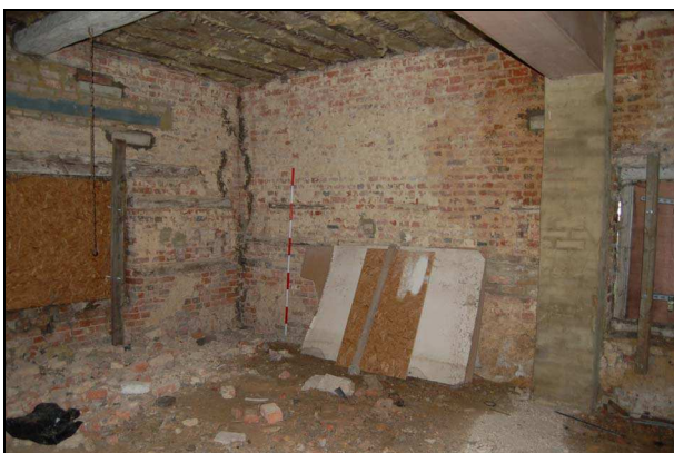
Plate 17: Room G1: northwest corner
