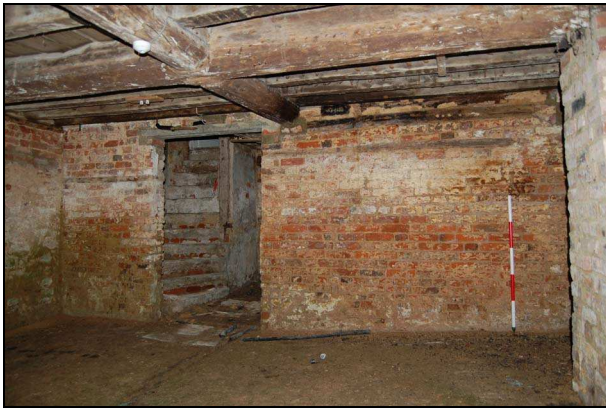
Plate 13: Cellar C2: east wall
