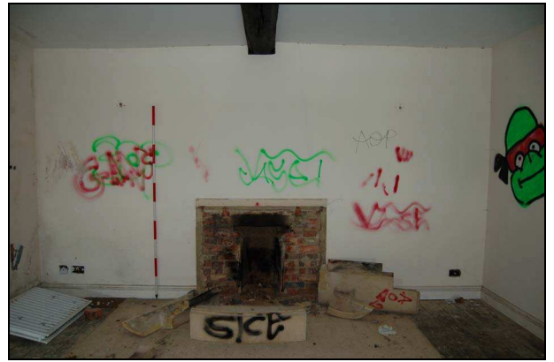
Plate 38: Room G5: west wall
