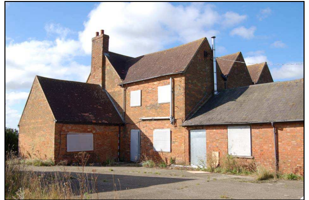
Plate 4: East elevation, north range
