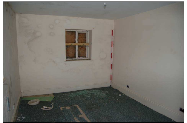
Plate 58: Room F8: north wall
