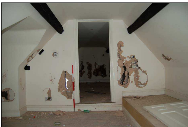
Plate 65: Room S2: east wall
