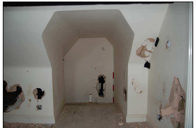
Plate 64: Room S2: south wall
