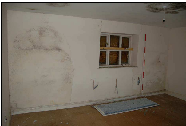
Plate 53: Room F5: north wall
