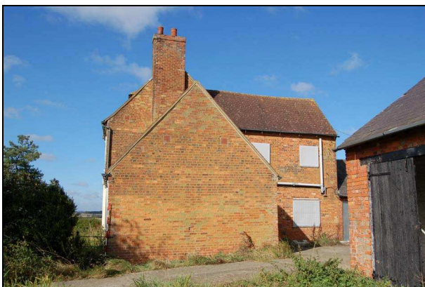
Plate 5: East elevation, south range
