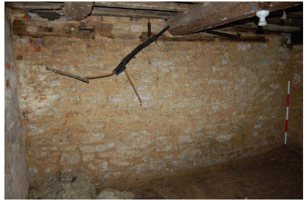
Plate 8: Cellar C1: east wall
