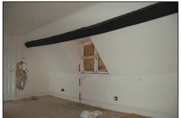
Plate 70: Room S3: south wall
