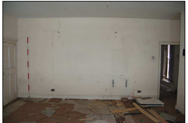
Plate 28: Room G3: north wall
