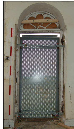
Plate 32: Room G4: door
