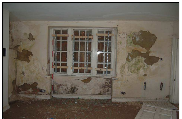
Plate 30: Room G3: south wall
