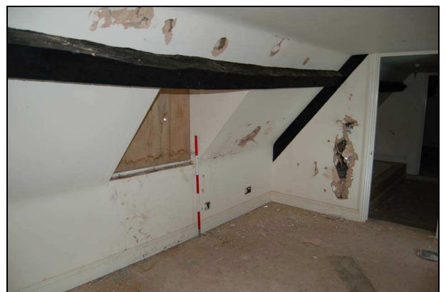
Plate 60: Room S1: southwest corner
