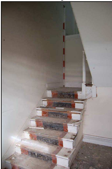
Plate 33: Room G4: staircase
