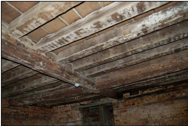
Plate 15: Cellar C2: ceiling looking northeast
