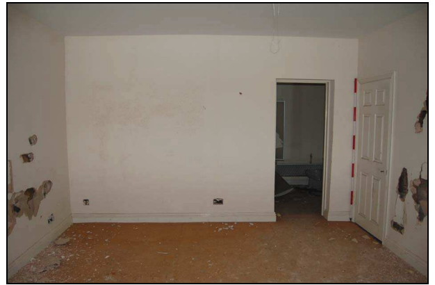
Plate 50: Room F3: north wall
