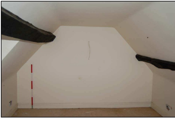
Plate 67: Room S3: west wall
