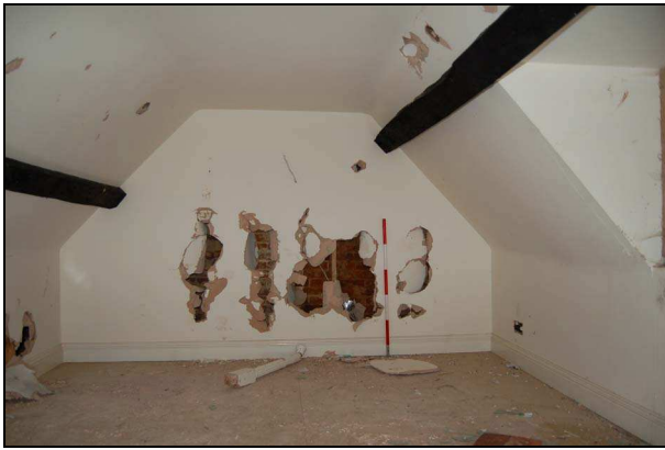
Plate 61: Room S1: east wall
