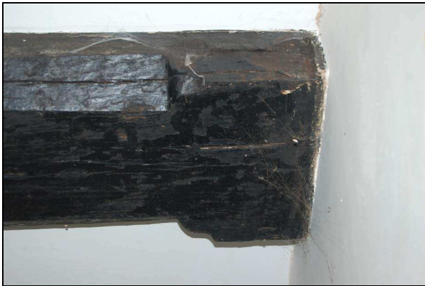
Plate 31: Room G3: Lamb's Tongue Chamfer Stop
