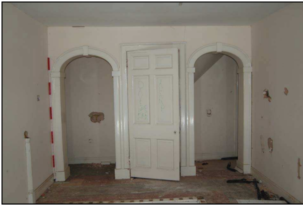
Plate 43: Room F1: north wall
