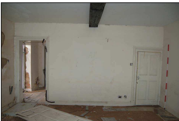
Plate 29: Room G3: west wall
