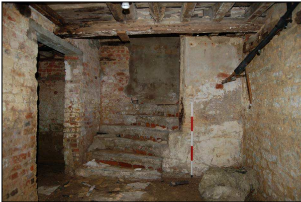
Plate 7: Cellar C1: north wall
