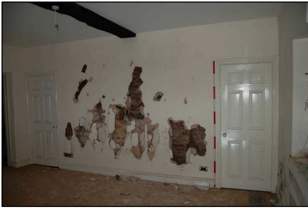
Plate 49: Room F3: east wall
