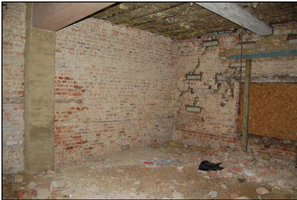
Plate 21: Room G1: southwest corner
