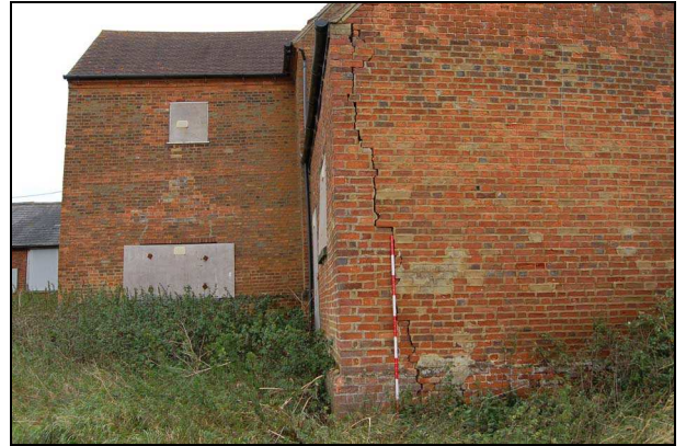
Plate 2: West elevation, north range
