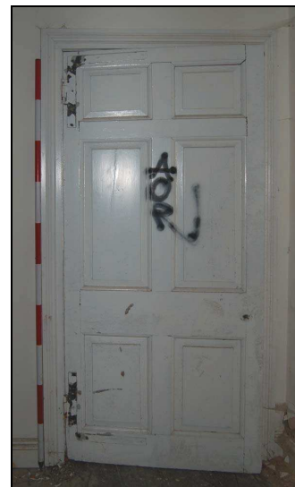
Plate 40: Room G5: door with L hinges
