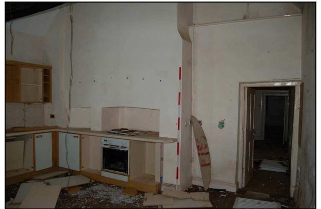
Plate 22: Room G2: west wall
