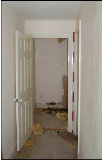
Plate 55: Room F6: looking north
