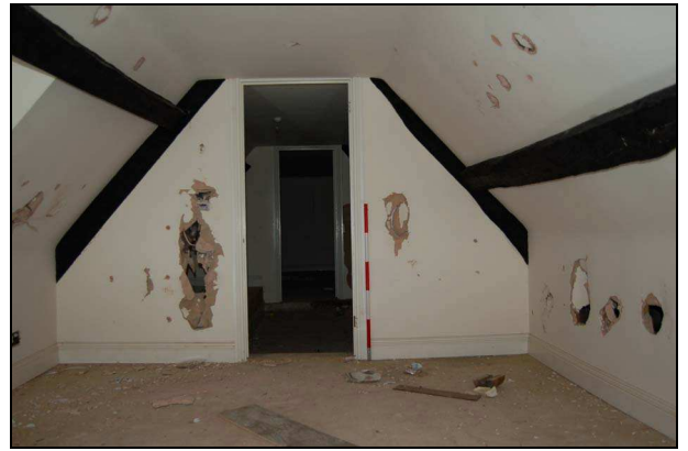
Plate 62: Room S1: west wall
