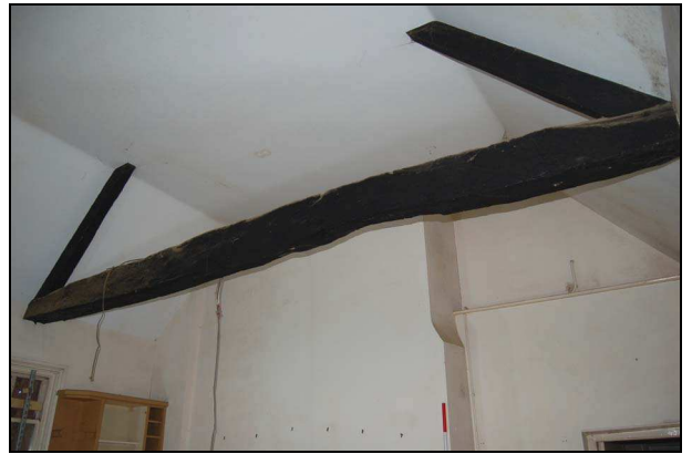
Plate 26: Room G2: exposed truss
