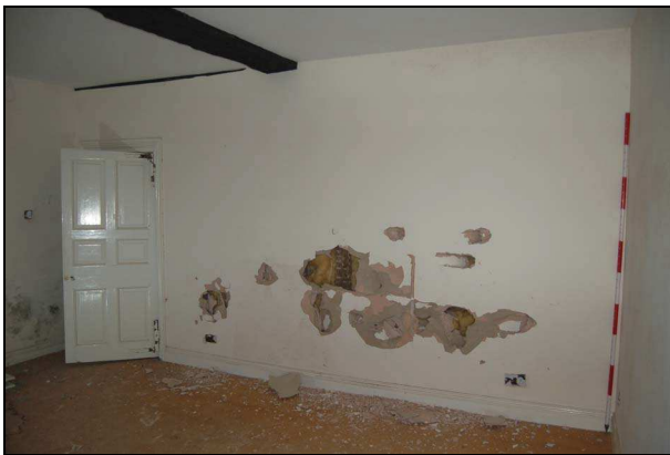
Plate 51: Room F3: west wall
