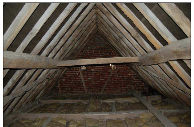
Plate 72: Roofspace viewed from Room S3
