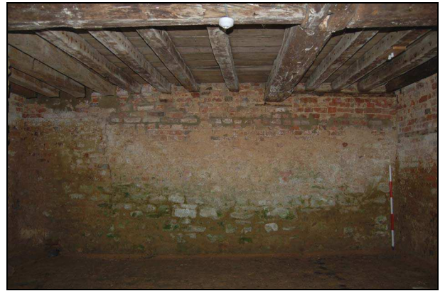
Plate 14: Cellar C2: north wall
