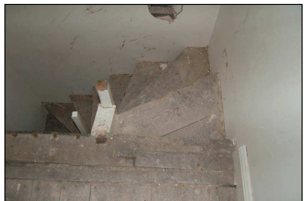
Plate 66: Room S2: stair & scarf joint
