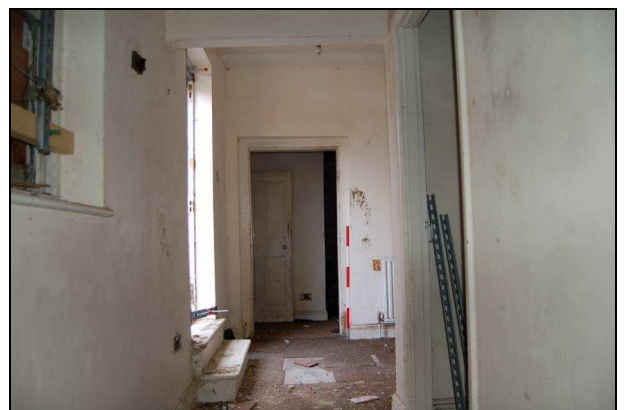
Plate 42: Room G6: looking south
