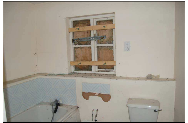
Plate 56: Room F7: east wall
