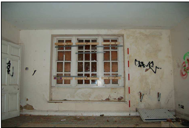
Plate 39: Room G5: south wall
