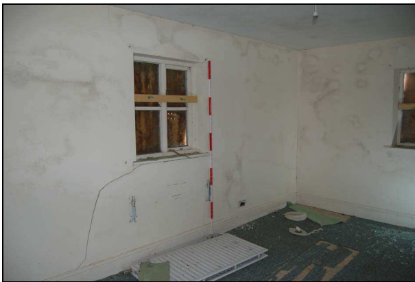
Plate 57: Room F8: northwest corner
