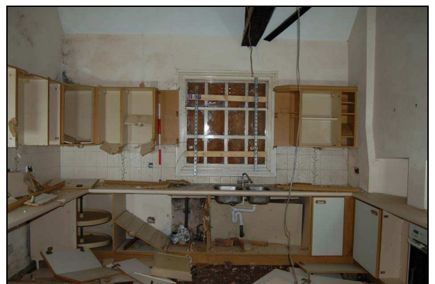
Plate 24: Room G2: south wall
