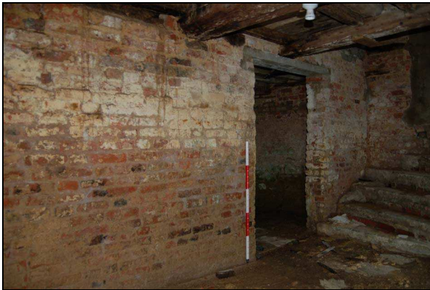
Plate 9: Cellar C1: west wall
