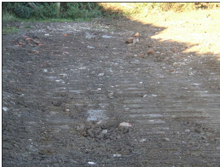
Plate 3: rubble spread by overgrown gate in Field C
