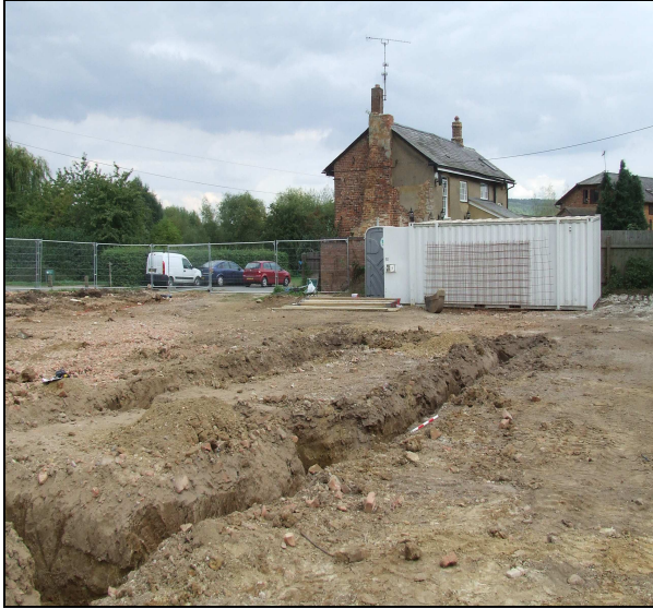
Plate 1: Looking NW towards Mill Farm House
