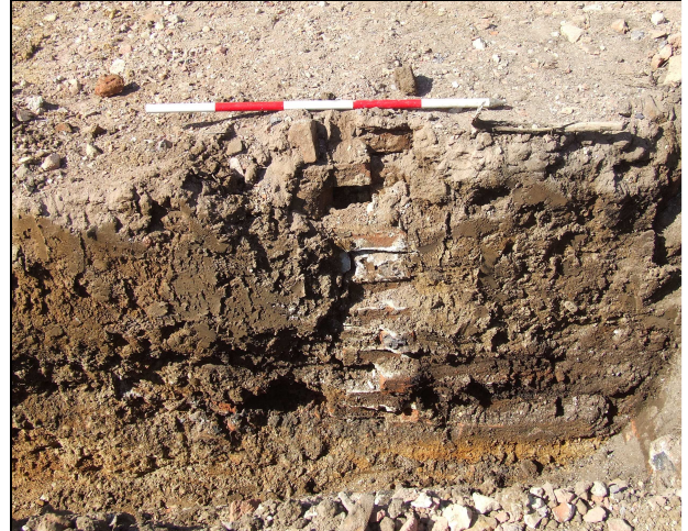
Plate 2: E facing section of footing trench showing wall foundations of recently demolished building 1m scale
