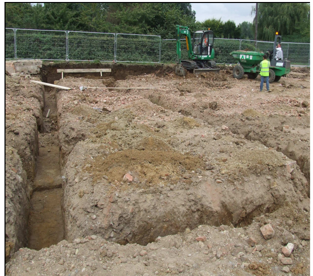
Plate 4: View NE across the footing trenches
