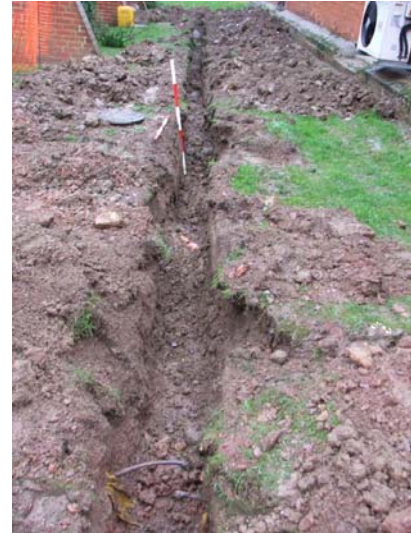
Plate 14: Trench I, facing S
