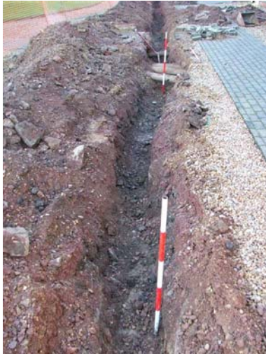
Plate 7: Centre of Trench H showing services, facing W
