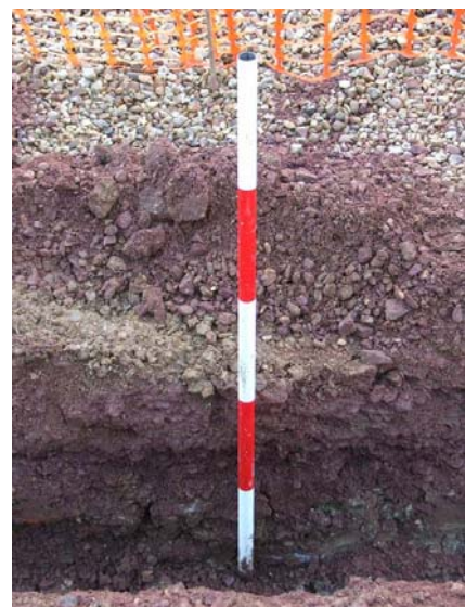
Plate 6: Trench H-East end section, facing NW
