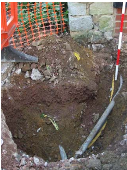
Plate 3: Test pit B1, facing N
