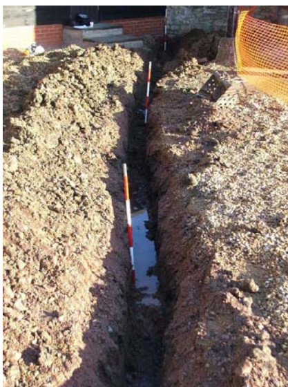
Plate 5: Trench H East end, facing NE.
